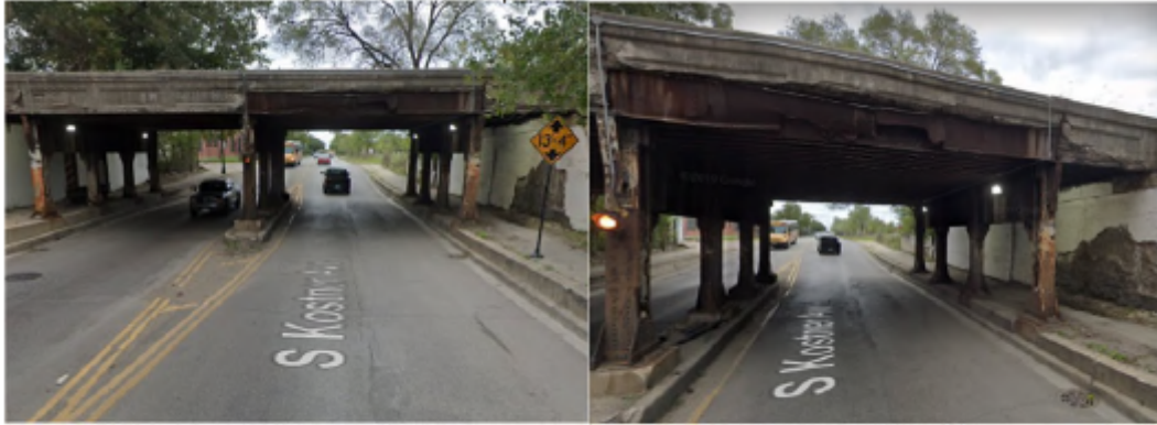
Kostner Facing northbound at CSX Viaduct
