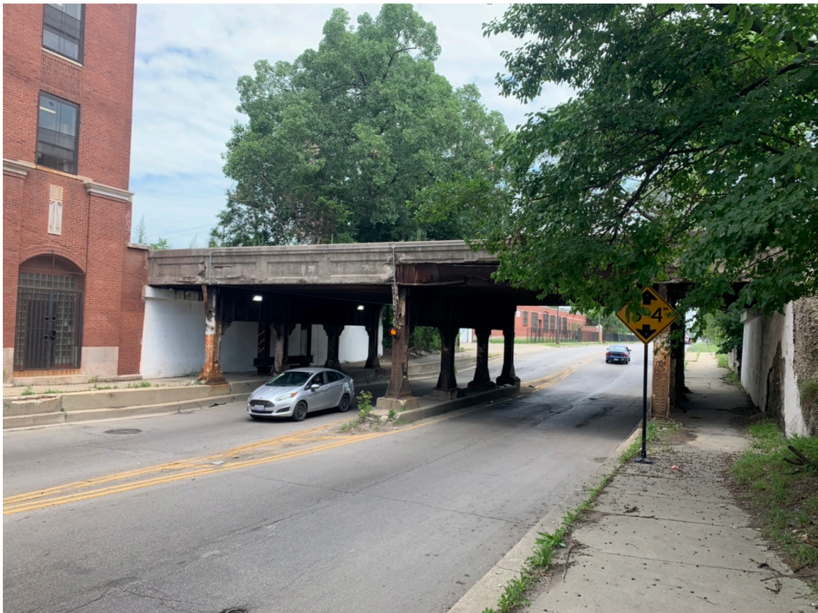
Kostner Avenue Viaduct looking north
