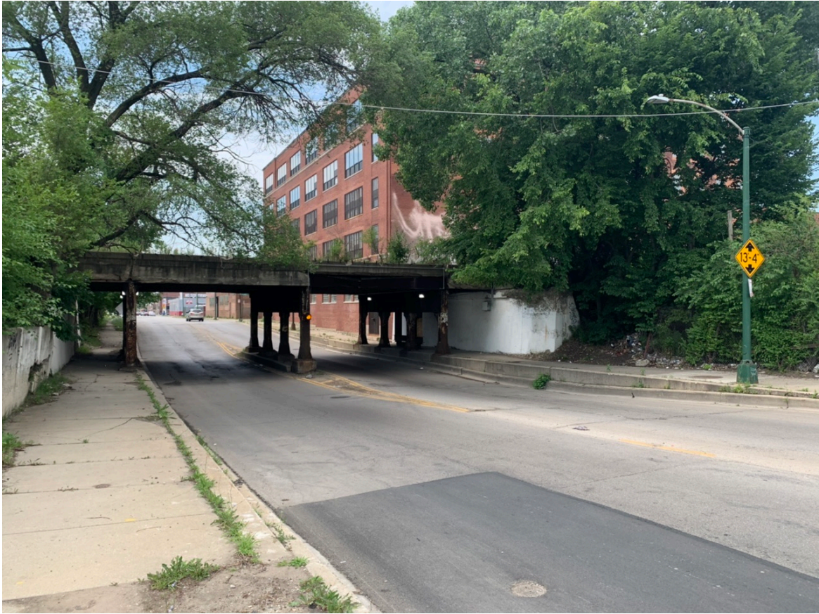
Kostner Avenue Viaduct, looking south
