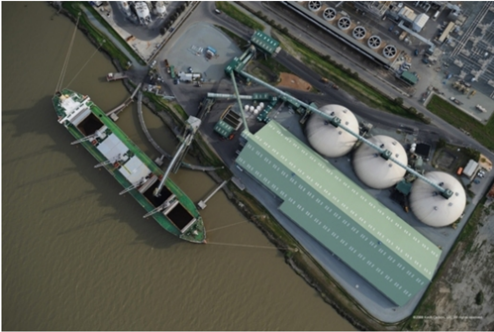
Koch Carbon's transfer facility in the San Francisco Bay area.
