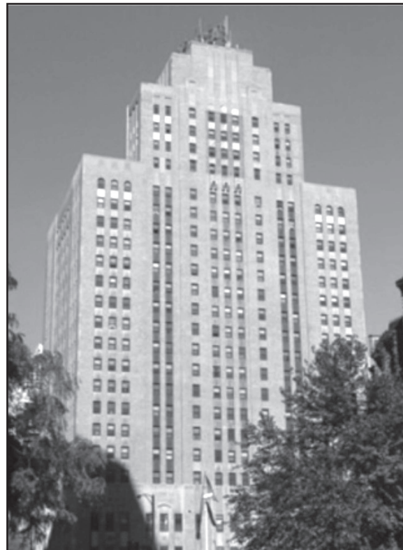
The City is providing $2.3 million in tax credits to enable the preservation of the largest SRO supportive housing facility in the Midwest while permanent financing is being arranged.
