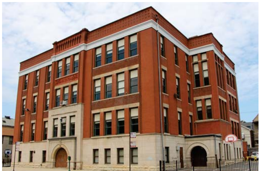
Peabody School, south elevation
