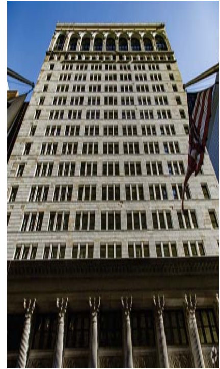
Commercial National Bank Building, west elevation
