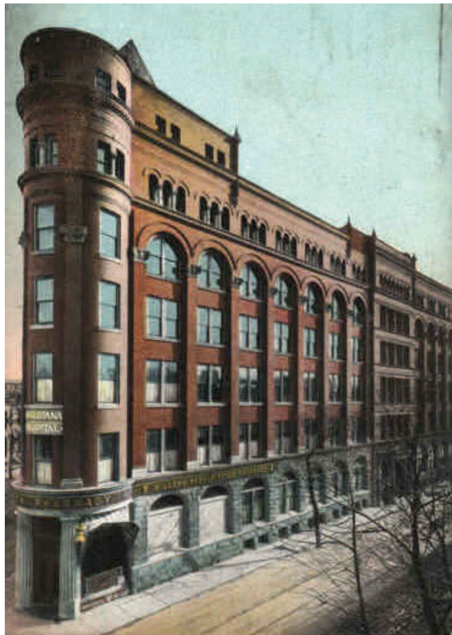
Hallberg designed three hospitals (early buildings for Swedish Covenant Hospital, Augustana Hospital and Woman's Hospital) as well as two medical college buildings for the Polyclinic Medical College and the Woman's Medical College. Top: A lithograph from the early 1890s showing several Chicago hospitals and medical college buildings, including the Woman's Medical College (marked by arrow), originally on the Near West Side on S. Wolcott (demolished). Right: Hallberg's building for Augustana Hospital, located at the intersection of N. Lincoln and N. Cleveland avenues (demolished).
