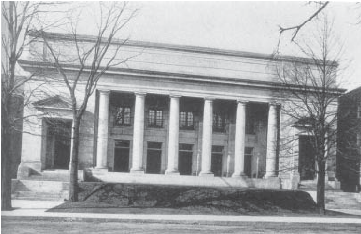
Beman designed many Christian Science church buildings, including six in Chicago, including (top) Second Church of Christ, Scientist at Wrightwood and Hampden in the Lincoln Park neighborhood; and (bottom) Fifth Church of Christ, Scientist on S. Dorchester Ave. in the Kenwood neighborhood.
