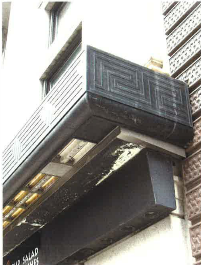
The photograph above shows one of the two building entrances modified between 1947 and 1951 with polished granite door surrounds as well as the steel and glass storefronts. The photograph at left shows the black metal soffit installed sometime between 1918 and 1947 and cantilevered just above the first floor.
