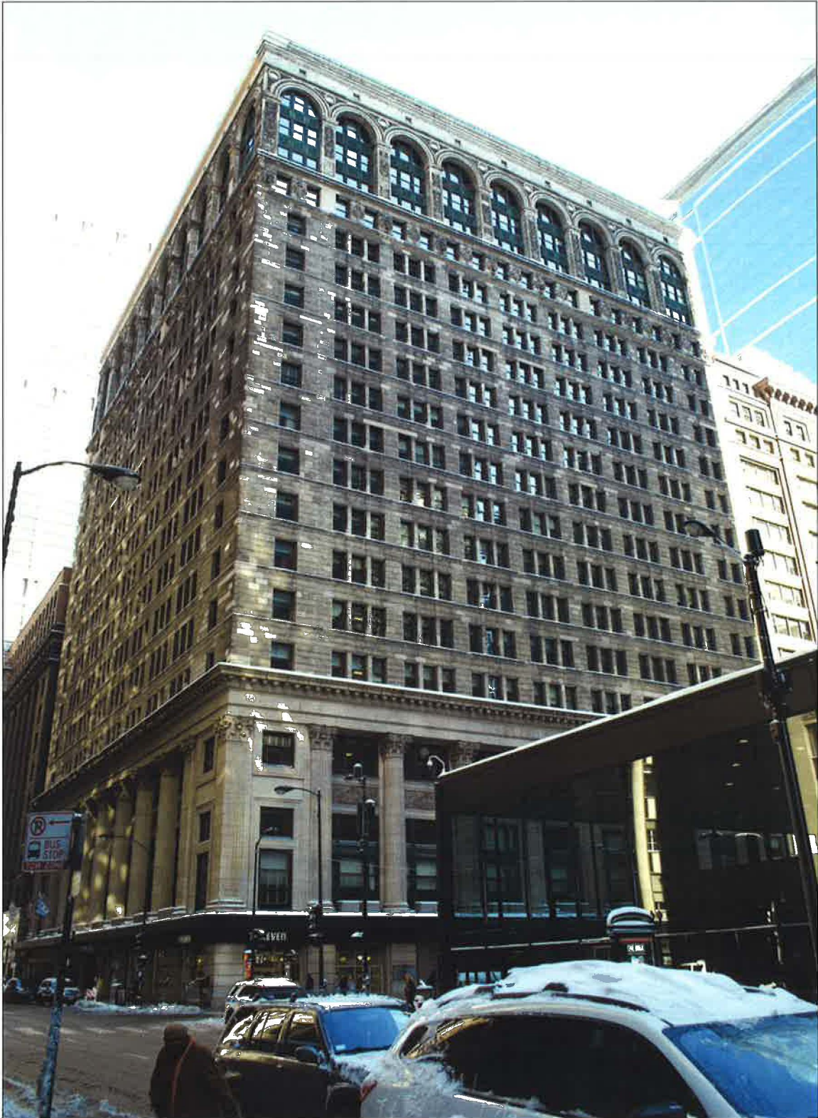
The Commercial National Bank Building/Edison Building is eighteen stories tall and clad entirely in architectural terra cotta produced by the Northwestern Terra Cotta Company. The tripartite composition, typical of early 20th-century skyscrapers, divides the building into a distinct base, mid-section, and top. The building is ornamented on all levels with a variety of Classical Revival design motifs.
