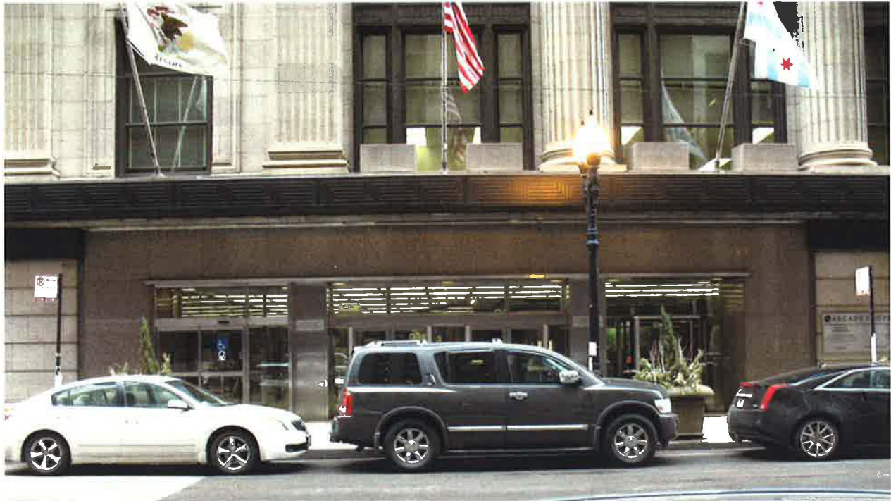
The photograph above shows one of the two building entrances modified between 1947 and 1951 with polished granite door surrounds as well as the steel and glass storefronts. The photograph at left shows the black metal soffit installed sometime between 1918 and 1947 and cantilevered just above the first floor.
