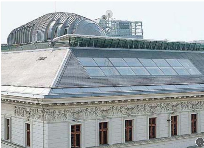
While this building is actually new construction, the treatment of the top of the building illustrates one approach to new additions. This rooftop portion of the building is set back from the facade to be minimally visible from the street. The addition's materials contrast with that of the lower, more visible portion of the building, which is more typical of the character of the district. An exterior lighting scheme is used as a tool to unify the facades (photos a, b).
