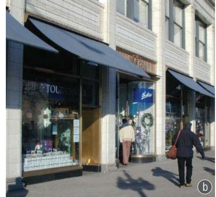
Retractable canvas awnings set within the bays of the building.
