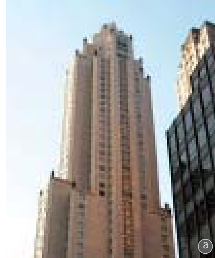
This tower has a distinct profile that is accentuated through multiple setbacks which continue to form a sculptural termination at the building top
