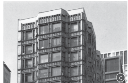
Reliance Building, missing cornice.
