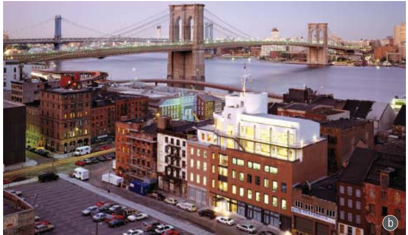
While this building is actually new construction, the treatment of the top of the building illustrates one approach to new additions. This rooftop portion of the building is set back from the facade to be minimally visible from the street. The addition's materials contrast with that of the lower, more visible portion of the building, which is more typical of the character of the district. An exterior lighting scheme is used as a tool to unify the facades (photos a, b).
