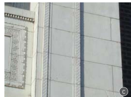
Terra cotta of the Santa Fe building
