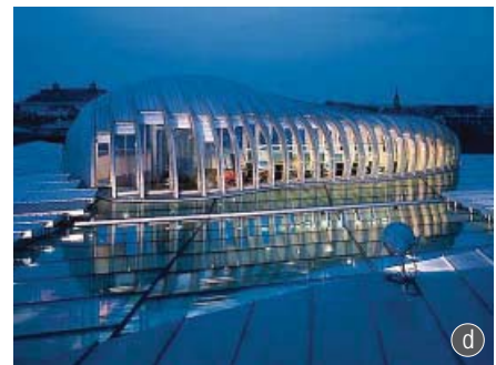
This sculptural rooftop addition is setback from the facade, minimizing its visibility from the street. The materials of this addition contrast the materials of the building below but maintain a scale consistent with the detailing of the same (photos c, d).
