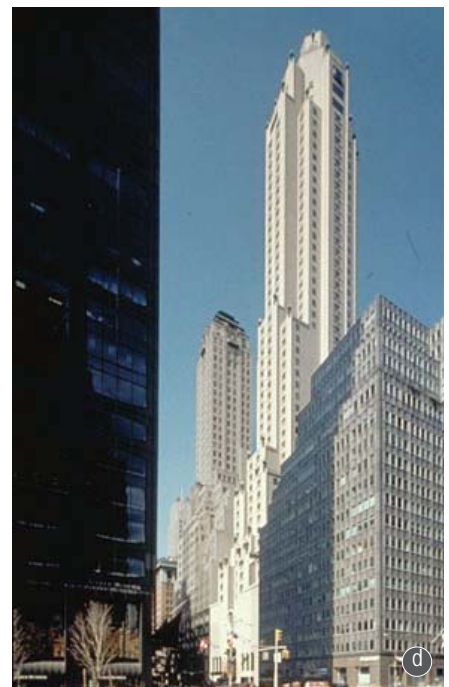
This tower represents an example of massing, upper level setbacks and facade design that reflect the characteristics of its surroundings. These design tools are also appropriate to the design of new construction for the Historic Michigan Boulevard District.
