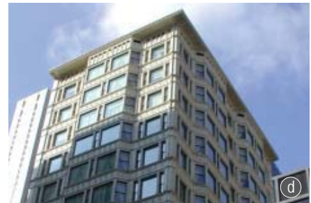
Reliance building with recreated metal cornice, 2001.
