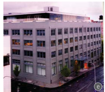
In the Northwest 13th Avenue historic district, this rooftop office addition is set back from the facade and is minimally visible from the street level (images c, d, e).
