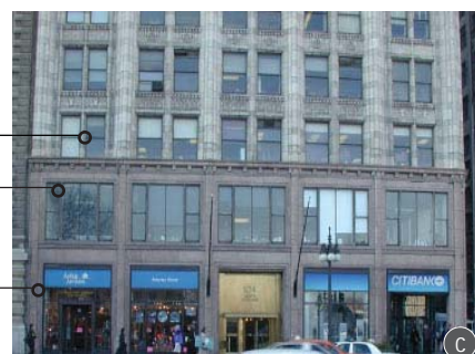
Monroe Building two-story base
