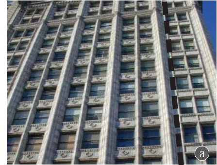
Verticality of Monroe Building mid section
