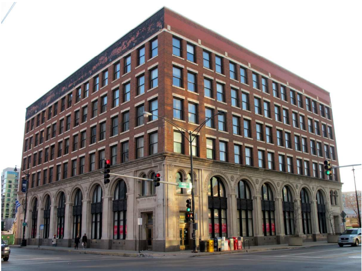
Floors three to six appear much as they did when the building was first built in 1911 as six story store and office building. In 1928 the limestone and granite base was added and a new banking hall was constructed on the interior.
