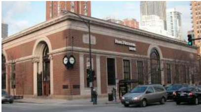
COSMOPOLITAN STATE BANK 801 N. Clark Street Date: 1920 Architect: Schmidt, Garden and Martin
