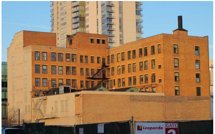
The less-visible west and south elevations (above) are common brick. The two story portion of the building in the foreground was originally the location of the separate Virginia Theater building. The theater was either completely demolished or radically altered to create the grand banking hall in 1928.
