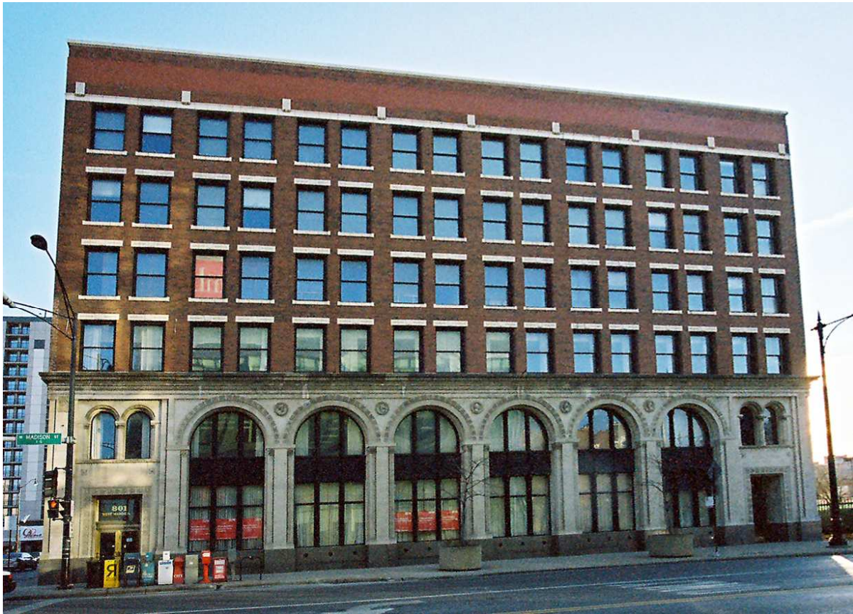
The Madison Street elevation as it appears today. Perkins, Fellows & Hamilton's 1928 limestone arcade transformed the exterior of the building's first two stories. With the exception of the lost cornice, floors three to six remain much as they appeared in 1911.
