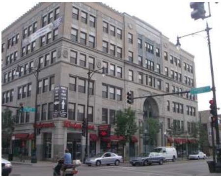
BELMONT-SHEFFIELD TRUST AND SAVINGS BANK 1001 W. Belmont Avenue Date: 1928-1929 Architect: John A. Nyden & Co.
