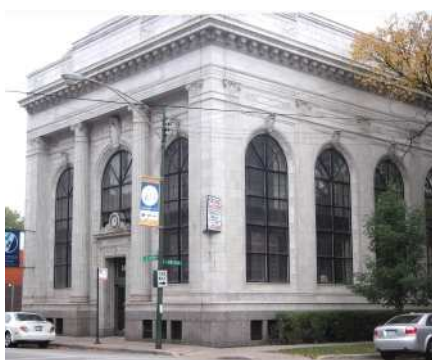
FULLERTON STATE BANK 1425 W. Fullerton Avenue Date: 1923 Architect: Karl M. Vitzthum
