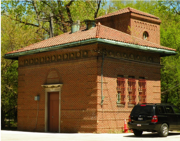
View of the Transformer Building — looking northeast.
