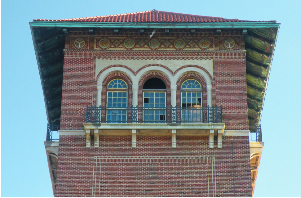
The Power House tower conceals a water tank and is decorated with copper eaves, clay tile roof, and mosaic tile frieze.
