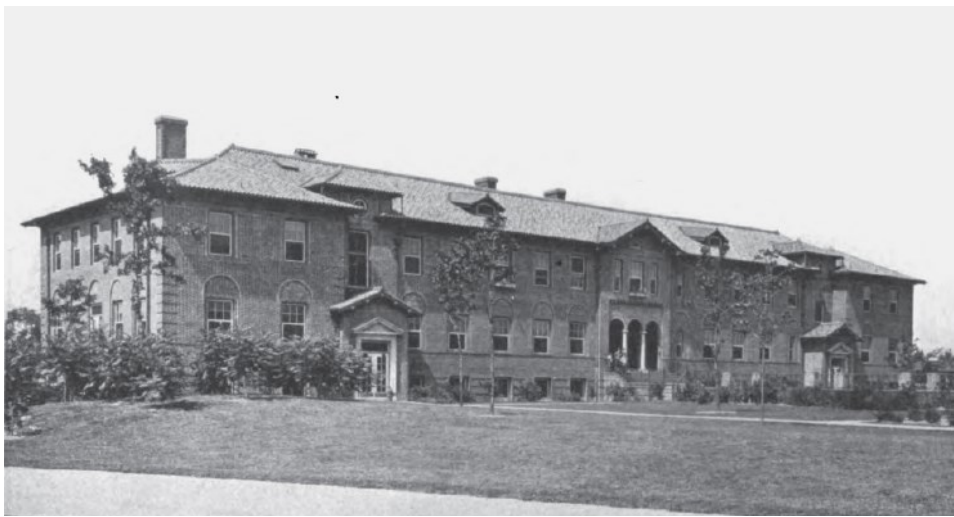
The Administration Building — looking northwest to the east elevation.
