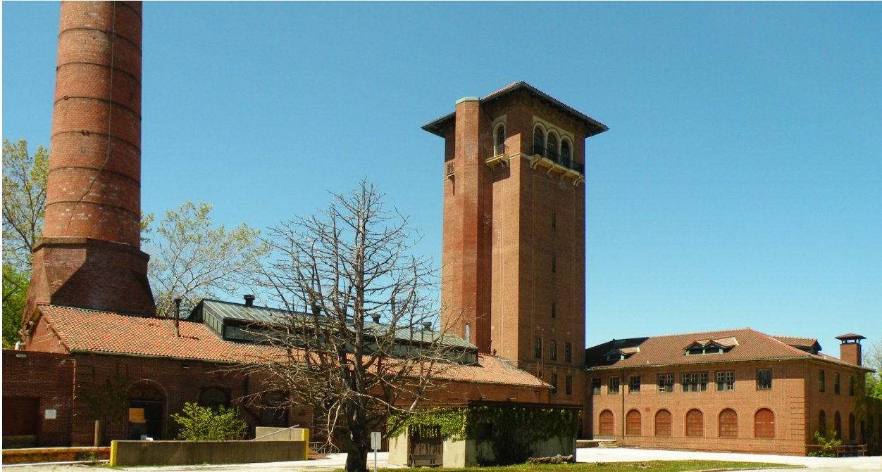
The Power House is comprised of a boiler wing (left), a tower (center), and a laundry section (right).
