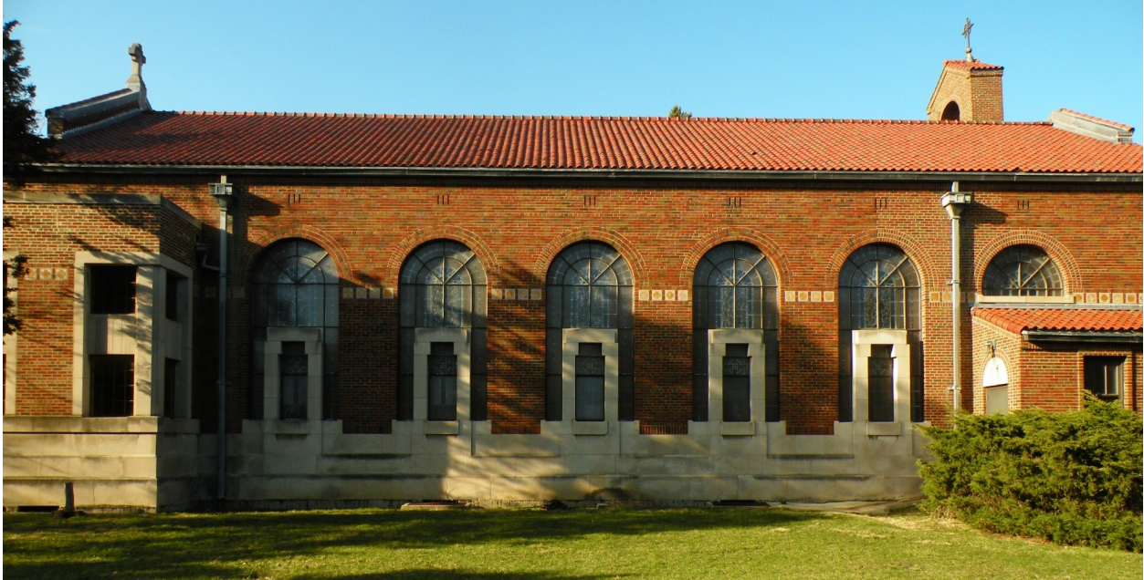
South elevation of the church showing fenestration and stone trim.
