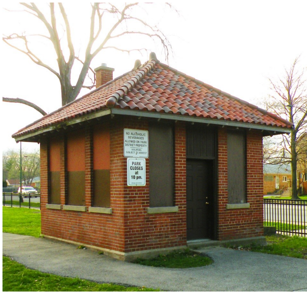
Above: South and east elevations
