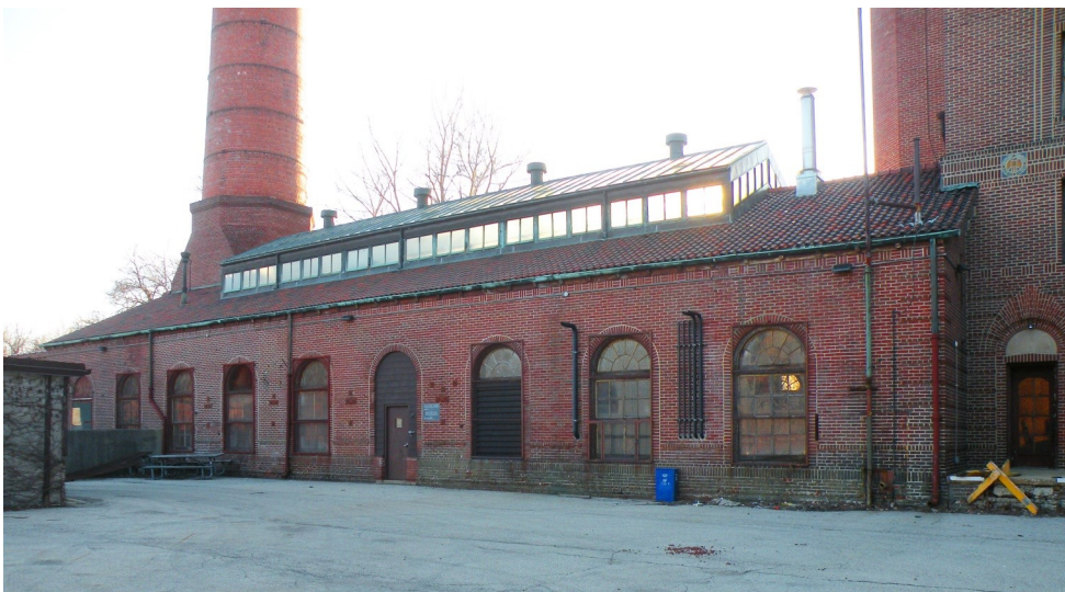
The boiler section of the Power House was extended in 1917 to accommodate larger boilers to provide heat to MTS.
