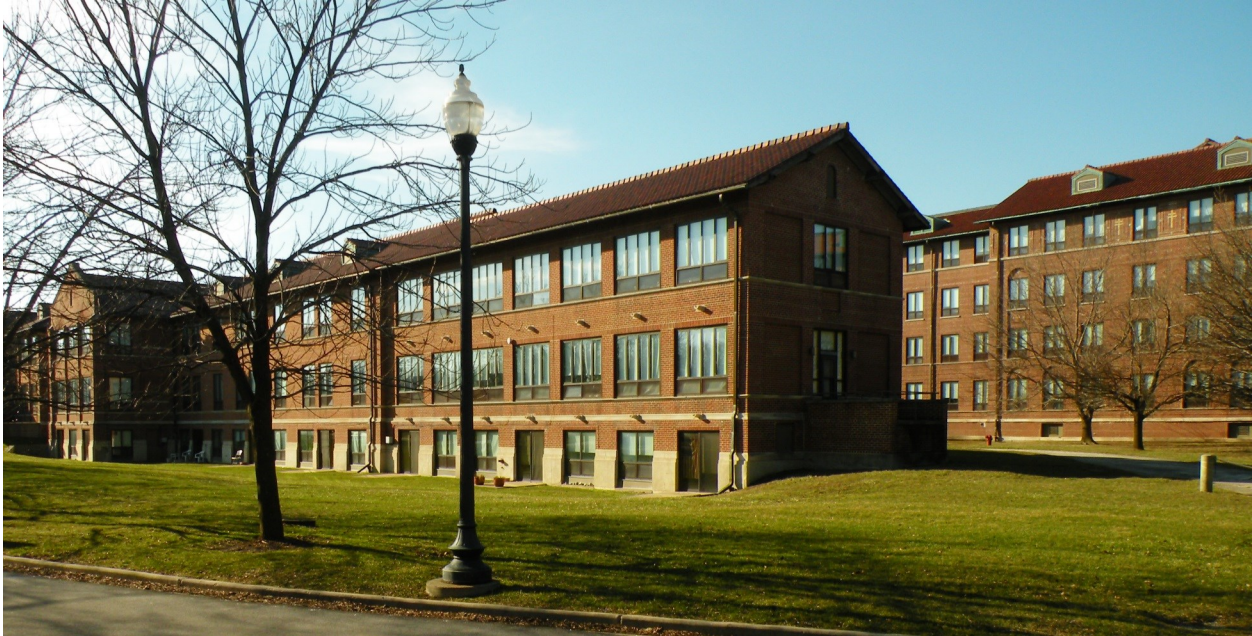
Looking northwest toward the Infirmiry Buildings. The open air section of the women's infirmiry wing is at center and the infirmiry annex is at right.
