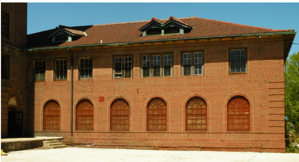
The laundry section had laundry facilities, housing for laundry workers, and, later, electrical generators in the basement.
