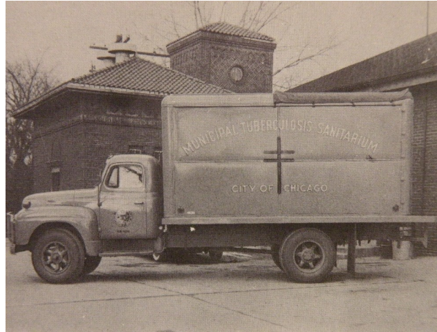
The Transformer Building and an MTS truck, c.1959. Chicago Public Library, Municipal Reference.
