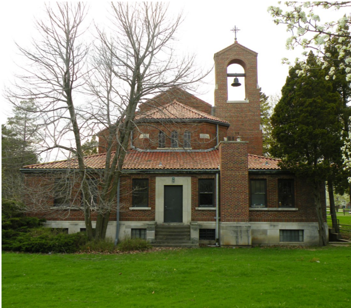
East elevation of the church showing the bell tower.
