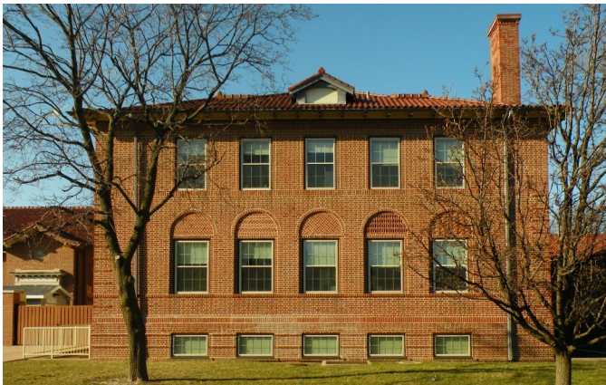
South elevation of the Service Building. Showing tympanum with different brick patterns.
