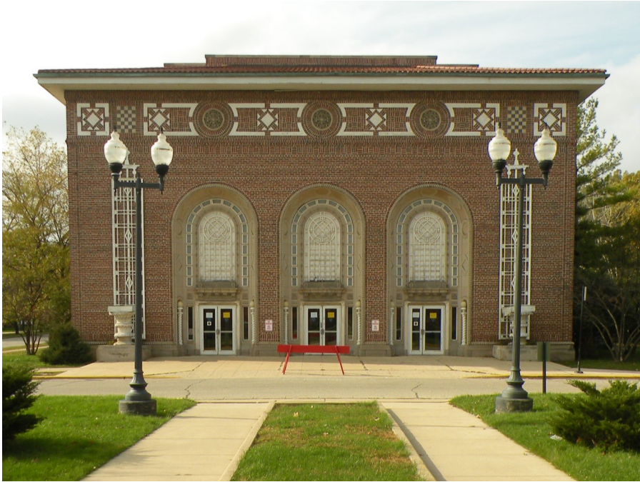
Main east elevation of the Auditorium Building.
