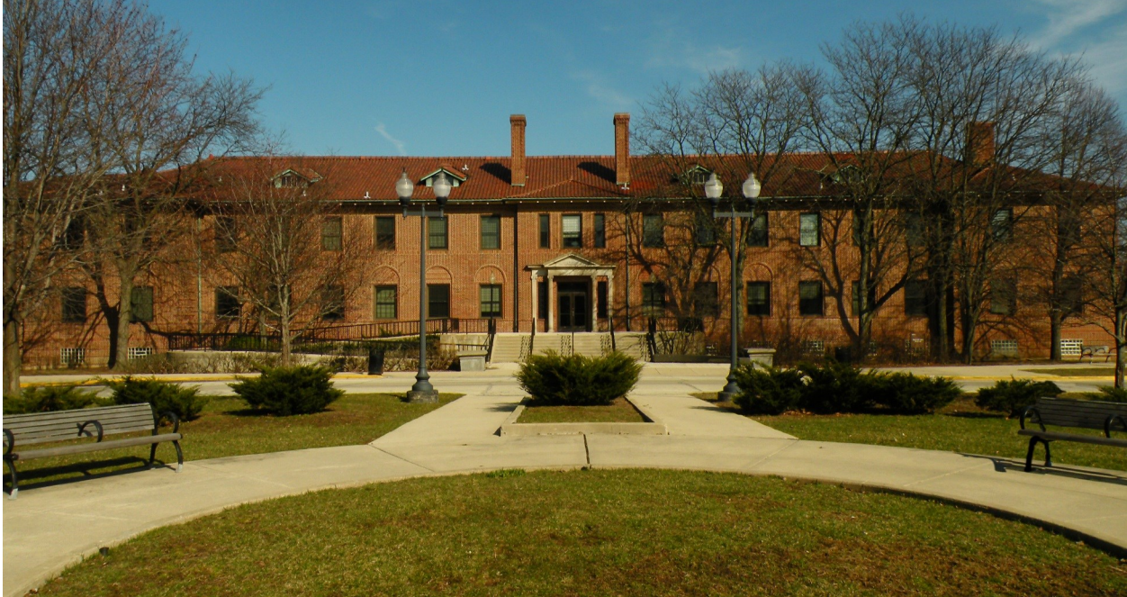
Main west elevation of the Administration Building.
