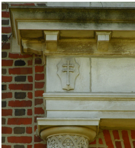
Cross of Lorraine carved in limestone on the Men's Dining Hall portico.
