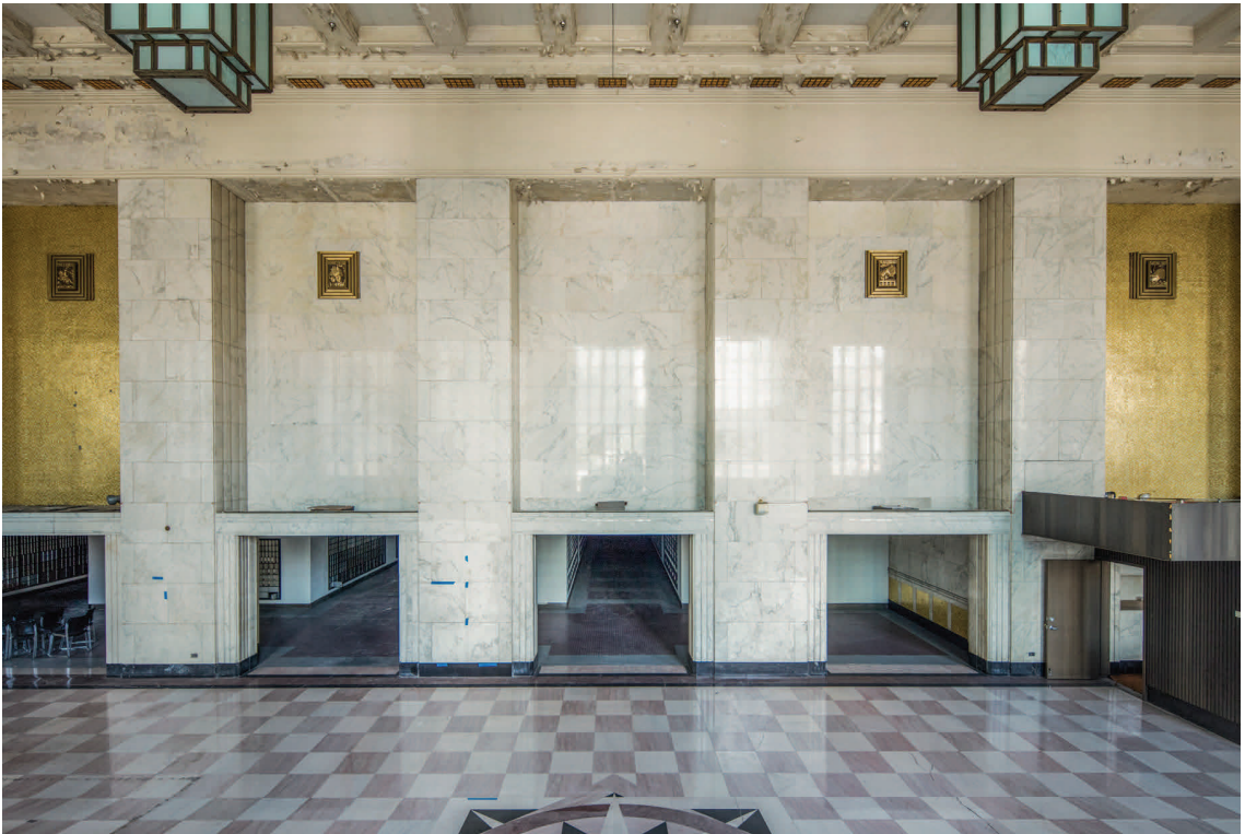
Photographs of the building's main lobby with its white-marble walls, polychromatic-stone floor, gold glass-mosaic details, and rectilinear metal-and-glass light fixtures (Tom Rossiter, photographer).
