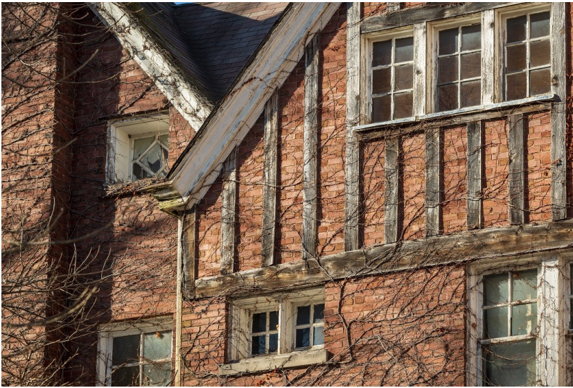
Above: The medieval-inspired half-timbering on the end of the north gable and the varied sizes, types and configurations of the windows are inspired by the Queen Anne style.
