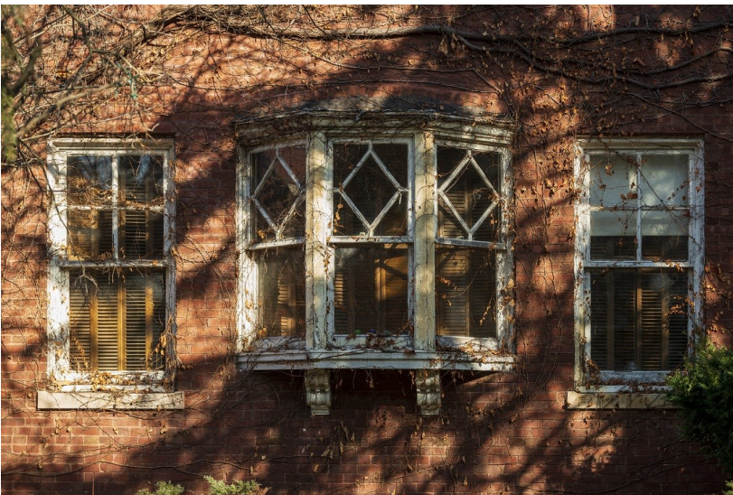
Above: Window types include this oriel window supported by brackets at the south elevation. The diamond motif is picked up again here.
