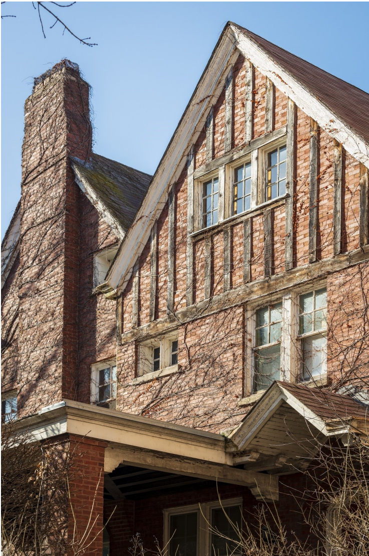
Three extant exposed rafter ends support the portico over the front door. (Photo by Patrick L. Pyszka)
