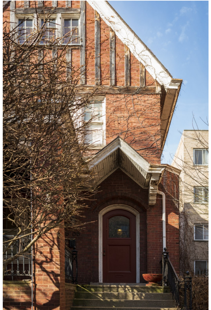
The recessed plane of the arched entry contrasts with angular, projecting, bracketed portico on the east elevation. (Photo by Patrick L. Pyszka)
