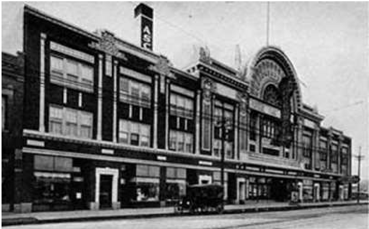
A circa 1920 photograph of the Portage Theatre compared with the current photo on the facing page shows that the building retains the majority of its architectural features.
