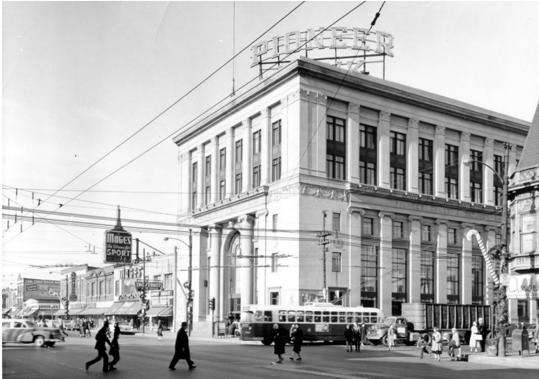
Above: looking northwest from North Avenue toward the Pioneer Bank at Pulaski, circa 1960. (Source: North and Pulaski Historical Society)
