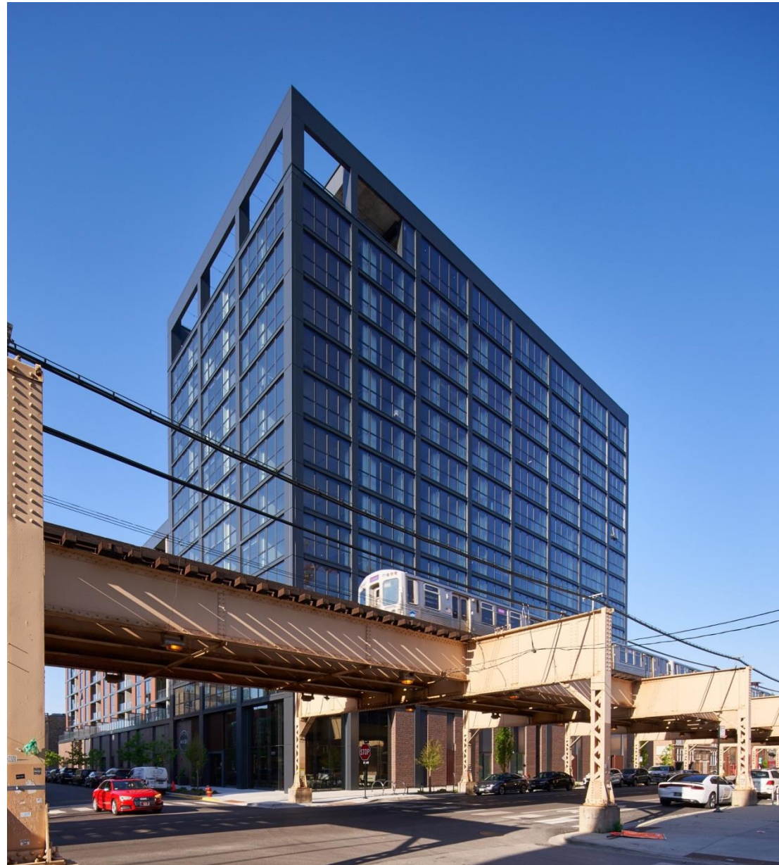
OVERALL BUILDING VIEW FROM STREET LOOKING SOUTHEAST
