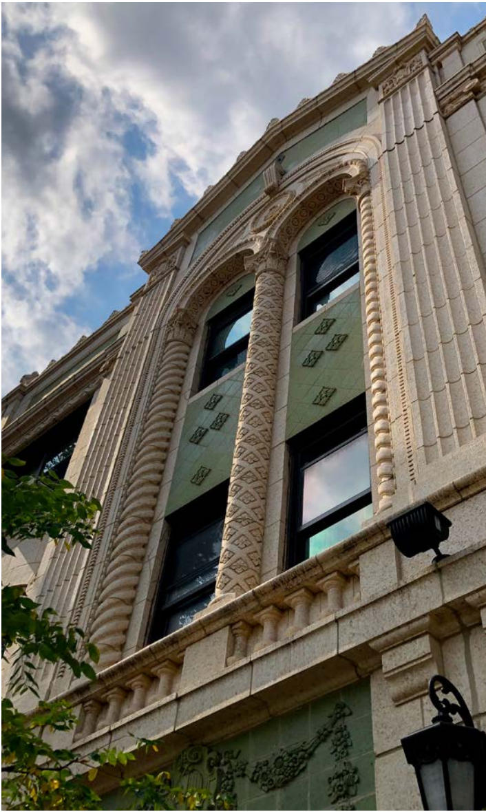
Historic Façade and Massing
