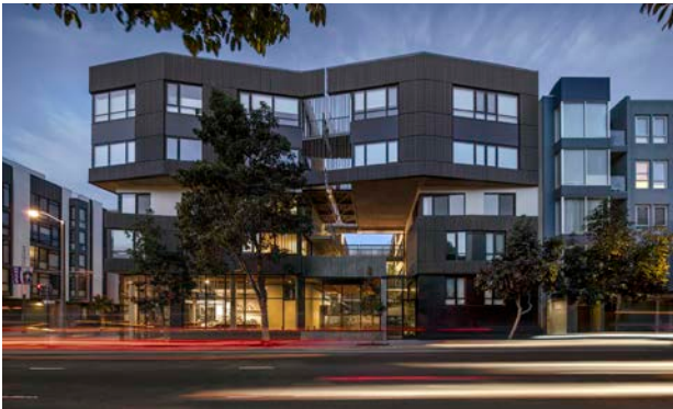
Source: 400 Grove, San Francisco, CA (Fougeron Architecture)
