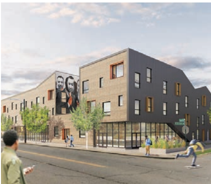
Source: Sawyer Apartment, Detroit, MI (ISA)
