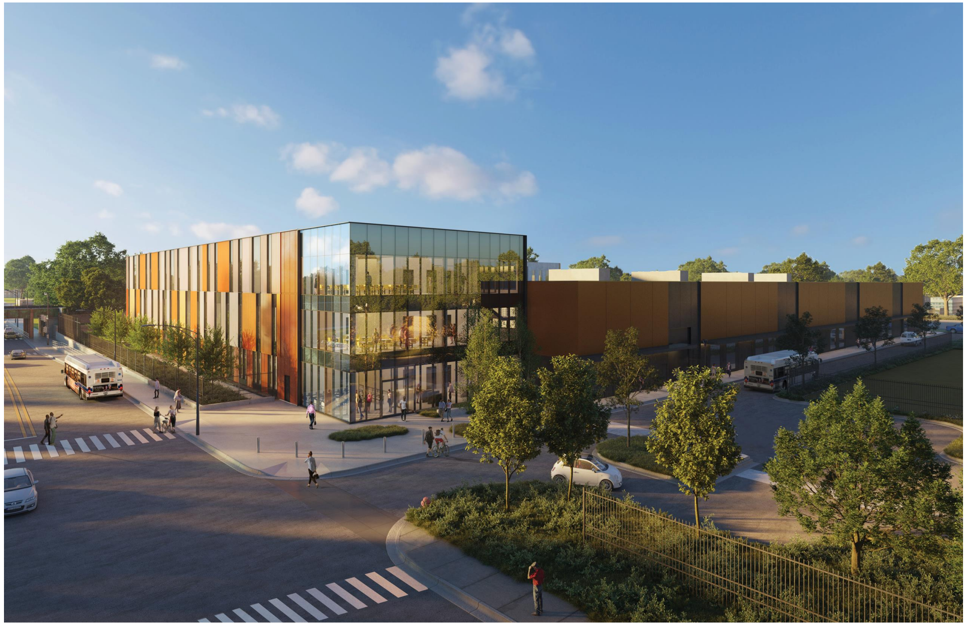
AERIAL VIEW FROM SW DIRECTION
