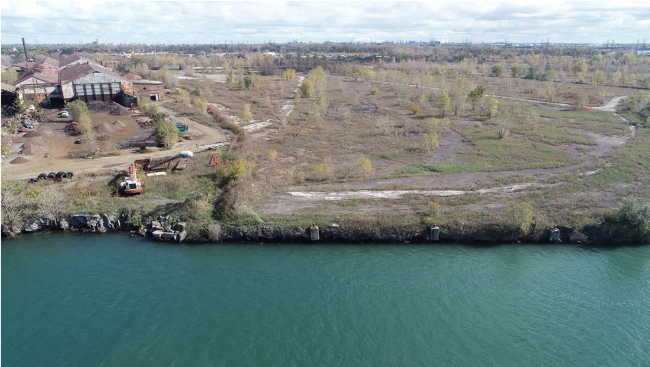
SITE CONTEXT – EXISTING CONDITIONS (VIEW FROM THE WEST)
