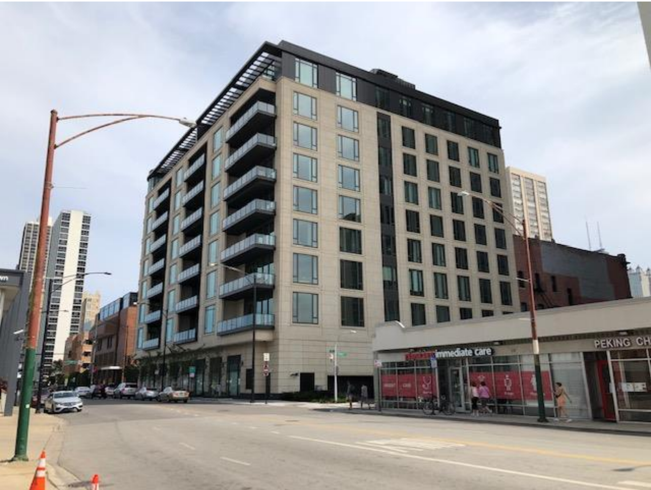
View looking East along North Avenue
