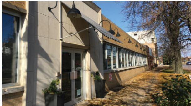
Awnings and canopies should be limited to the first floor and incorporate signage at the valance area. Open-ended awnings are the preferred standard, rather than boxed awnings.
