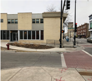
ADA Access- Lawrence and Ravenswood
