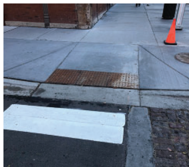
Typical Curb Ramps- Fulton and Morgan
