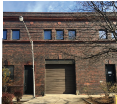
Loading and vehicle doors should maintain the size of the original opening and consistency with other openings in the building.
