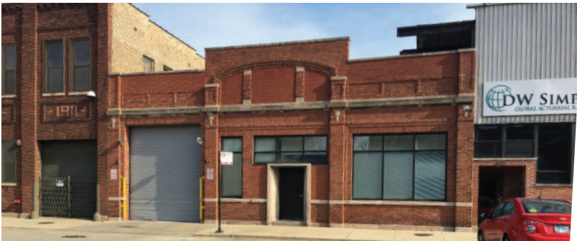
Decorative brick and stone features should be retained and repaired.
