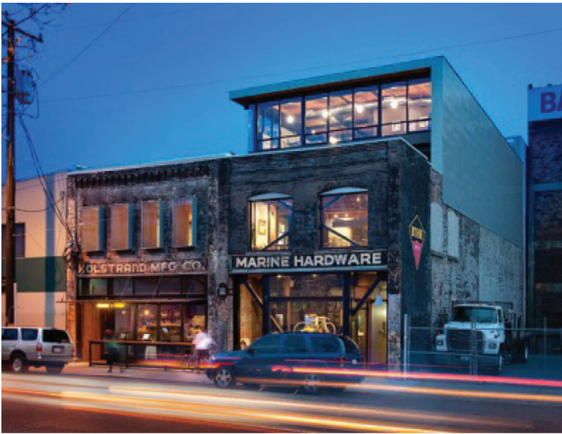
Example of an appropriate rooftop addition which is set back and has floor heights compatible with the existing building.
