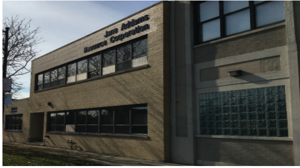
Continuous ribbon window openings are common in buildings from the 1930s and 1940s.
