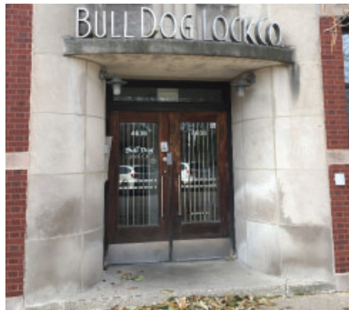
New doors should maintain the size and configuration of the original opening, including sidelights and transoms, and be appropriate to the character of the building.
