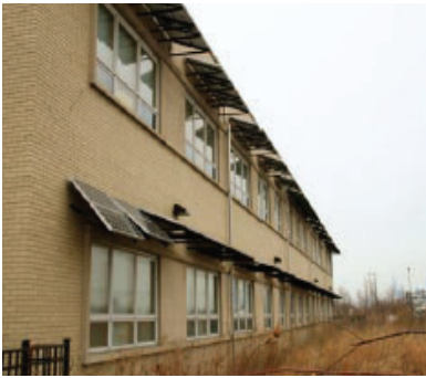
At the Chicago Center for Green Technology, solar panels serve a dual purpose, as they are used to generate electricity and are used as awnings above windows. This is an example of a non roof-mounted system.
