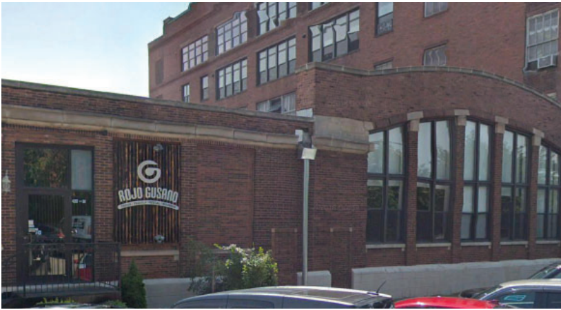
Example of an appropriate side and rear addition which incorporates durable materials including brick, limestone, and other compatible materials.
