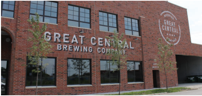
Example of a new light industrial building's orientation, massing, and scale. (221 N. Wood Street)
