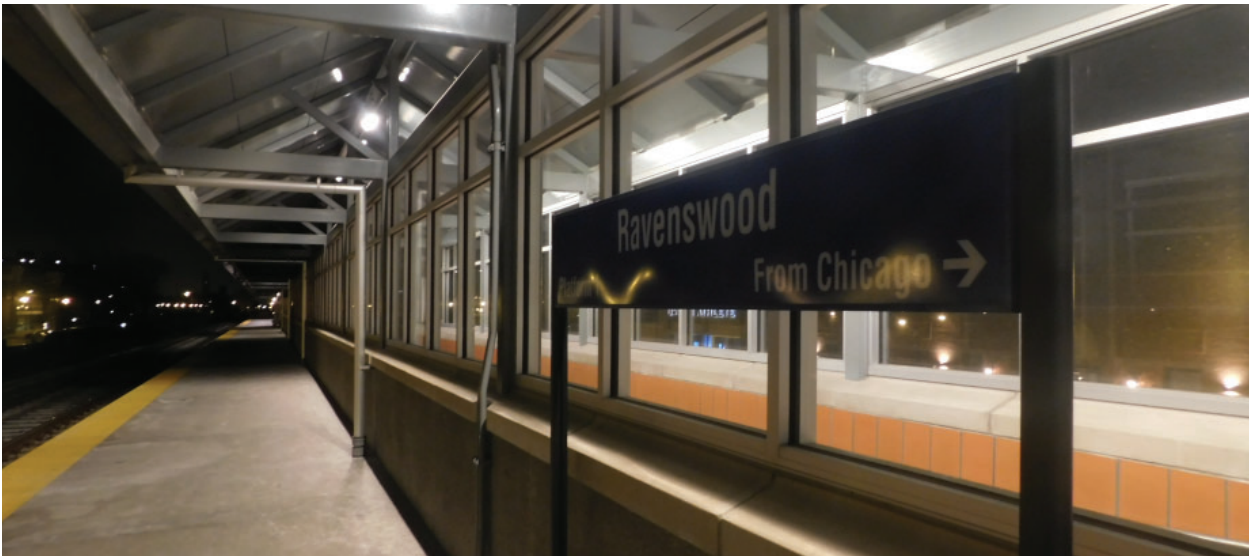
Metra Ravenswood Station, N. Ravenswood Avenue and W. Lawrence Avenue
