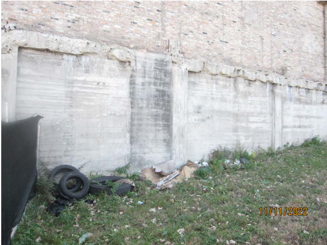
Photo 10: View of refuse and rubber tires near southeastern Site boundary and southern adjacent site building.
