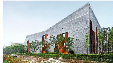
Sky Courts, Chengdu, China (2011)
