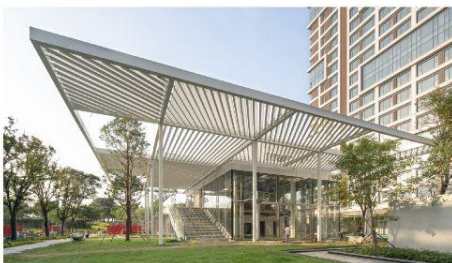
Helio House, Shenzhen, China (2021)
