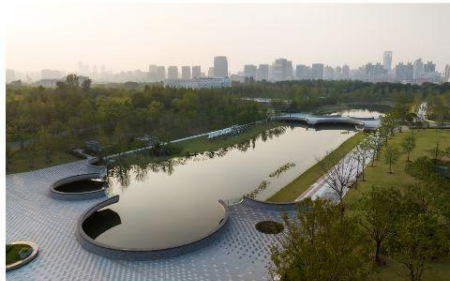
Moongate Bridge, Shanghai, China (2022)
