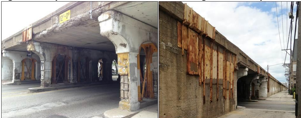
Figure 1. Hollywood Avenue Viaduct and Retaining Wall near Bryn Mawr Station
