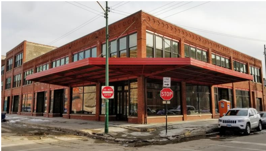
1113-1115 West Fulton Market (Fulton-Randolph Market District) Ward 27
