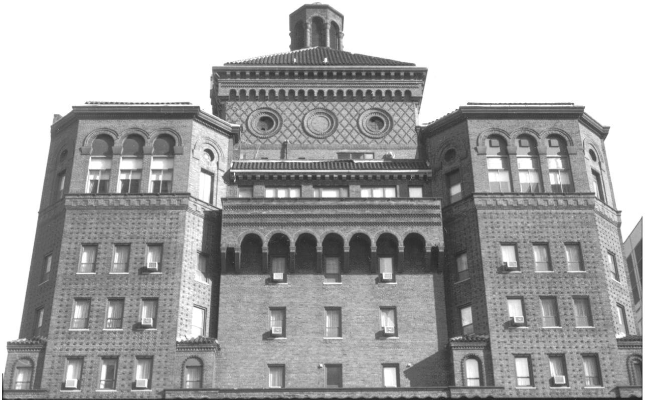
The top of the Allerton Hotel, as seen from the north, offers an assortment of setbacks and towers clad in patterned brick in a style meant to evoke the image of picturesque Italian towers.
