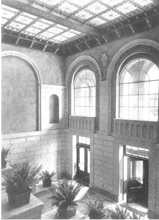
The building originally featured a two-story entrance foyer with a stained-glass ceiling and staircases leading to the second floor. Much of this space has been lost to subsequent remodeling.
