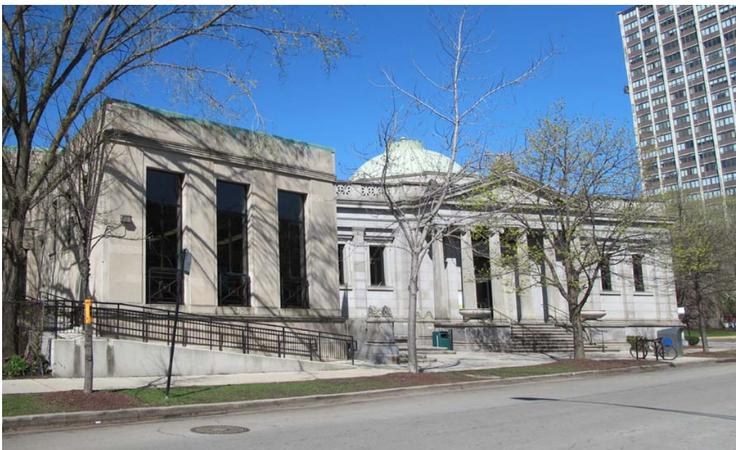
With federal funding from the Public Works Administration (PWA), an addition (shown at left in the photo above) was built to the south of the Blackstone Library in 1939.
