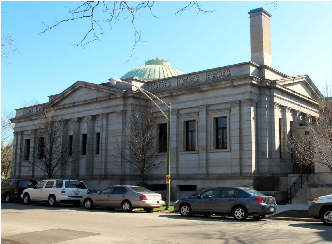
At top, the view of the primary front elevation of the building facing east. At bottom, the rear (west) elevation with its engaged portico; note also the use of similar pedimented porticos on the side elevations.
