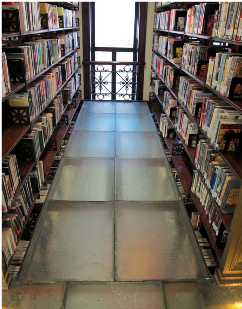
The shelving or “stack room” south of the rotunda with its mezzanine (top). The bronze medallion of Timothy B. Blackstone at the mezzanine railing (above) was created by New York sculptor William Couper. The structural slab glass floor of the mezzanine (left) allows light to reach the shelving on the lower level.
