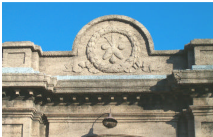
The Calumet Park Fieldhouse's Classical-style details are formed from cast concrete.
