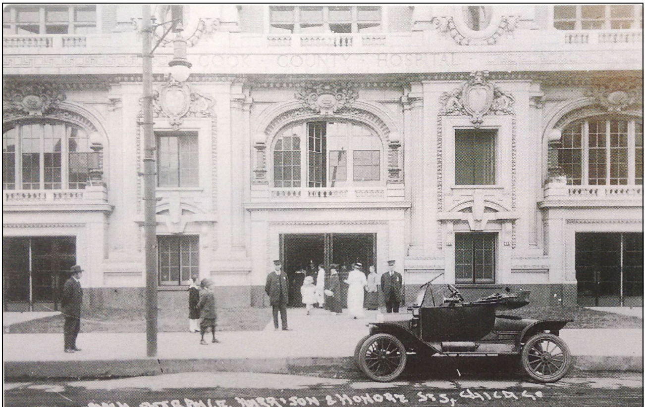
A historic photograph of the main entrance to the Cook County Hospital Administration Building soon after its opening in 1914 (from Chicago History Museum).
