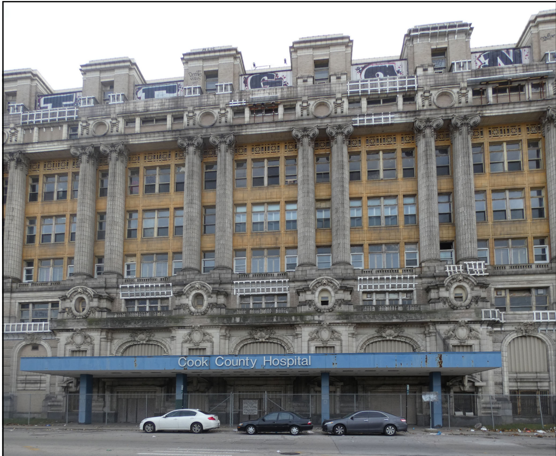
Bottom: Photograph of central section of building and main entrance, looking south.
