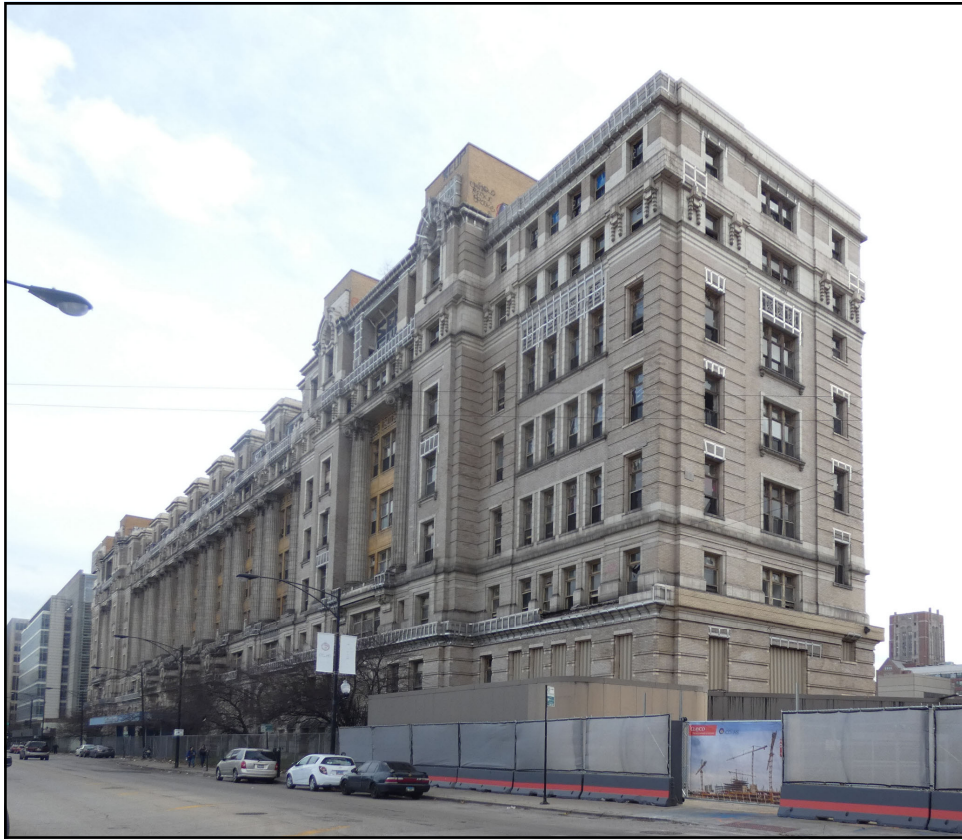
Current photographs of the Cook County Hospital Administration Building (courtesy MacRostie Historic Advisors)
