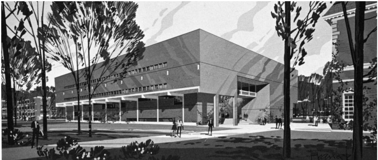
Above: Sawyer Library at Williams College (1975, Demolished), in Massachusetts. Designed during the energy crisis, Weese used passive cooling to eliminate the need for air conditioning. Left: Weese designed two-story study carrels at Sawyer to optimize space. Source: library.williams.edu
