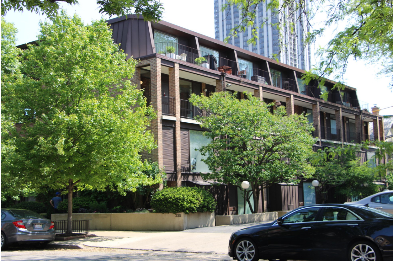
The rear elevation with projecting bays clad in standing-seam sheet metal that contain closets.
