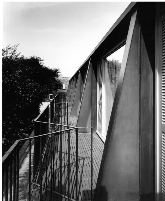
The mansard roof and balconies at the fourth floor. Source: Hedrich Blessing, 1962, Chicago History Museum, HB-25565.
