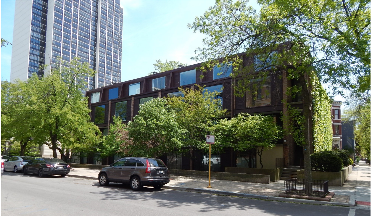
The front elevation of the Eugenie Lane Apartments. Chicago common-brick piers divide the facade into 7 bays. The recessed mansard roofline reduces the building's apparent height.
