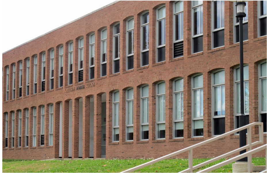
At the Northside Junior High School in Columbus, Indiana (1961), Ben Weese used a traditional system of brick arches and piers.
