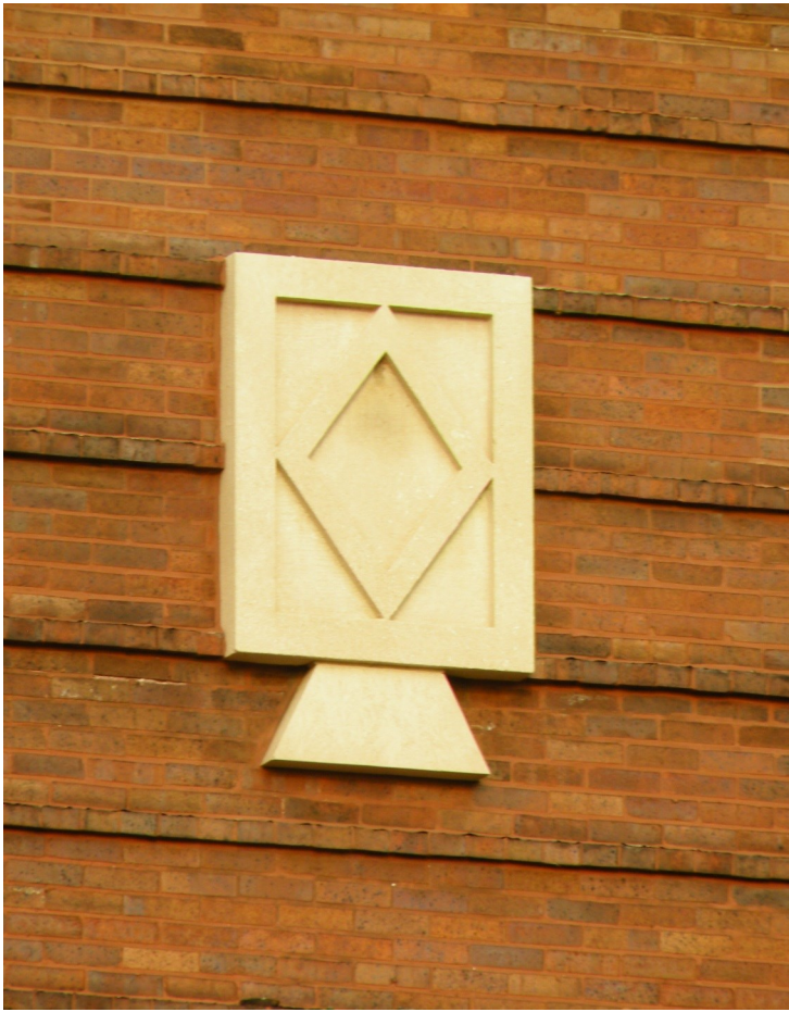
The walls of the Graeme Stewart Public School Building, both the original building and its addition, are finely detailed with brick rustication and geometric limestone plaques.
