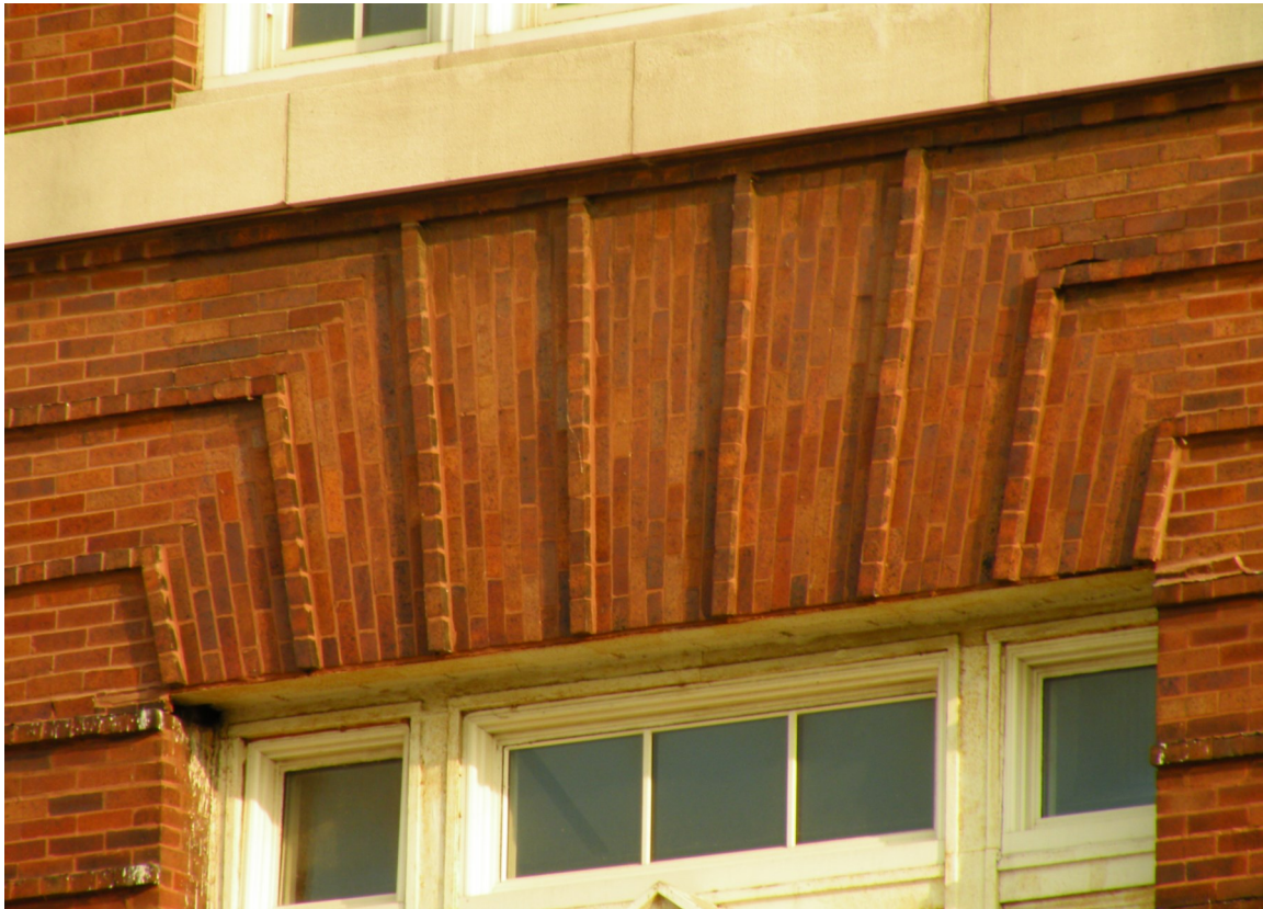
The walls of the Graeme Stewart Public School Building, both the original building and its addition, are finely detailed with brick rustication and geometric limestone plaques.
