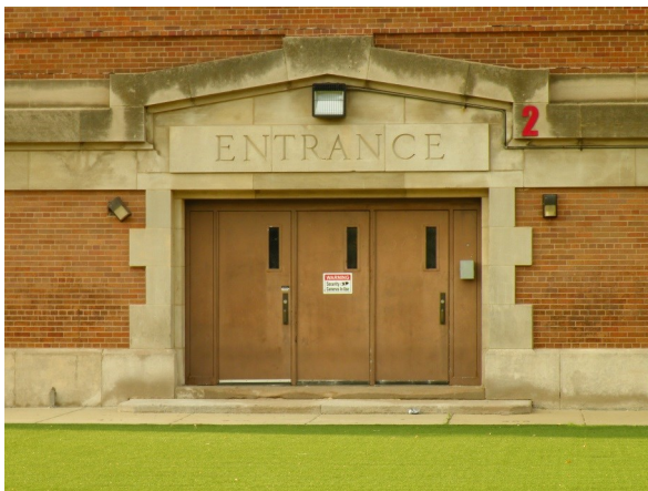
The 1940 south addition, although flat-roofed, is compatible in scale and design with the original school building, with rusticated-brick walls and contrasting gray limestone details. Top: A view of the addition from the southeast. Bottom left: The entrance to the addition. Bottom right: A photograph comparing the original building's hip roof and the flat roof and parapet of the addition.
