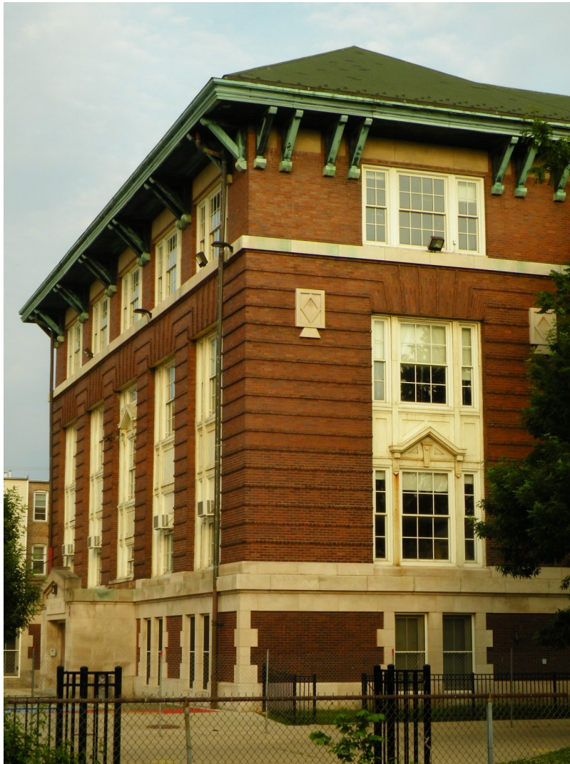
Left: A view of the building's northwest corner, showing the building's classical ornament, brick rustication, and grandly-scaled copper brackets. Bottom: The building's north entrance, with its abstract pediment and "BOYS ENTRANCE" inscription.
