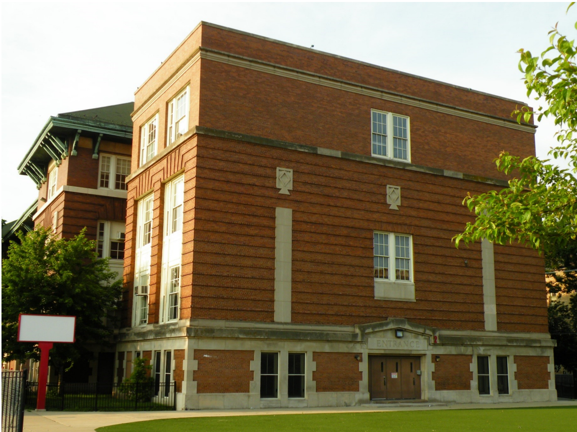
In 1940, a four-story addition was built at the south end of the Stewart Public School Building. It was designed by Board of Education architect John C. Christensen to mimic the original building in overall scale, building materials and detailing. Top: A postcard view of the addition in 1940 (source unknown). Bottom: A photograph of the addition in June 2016.
