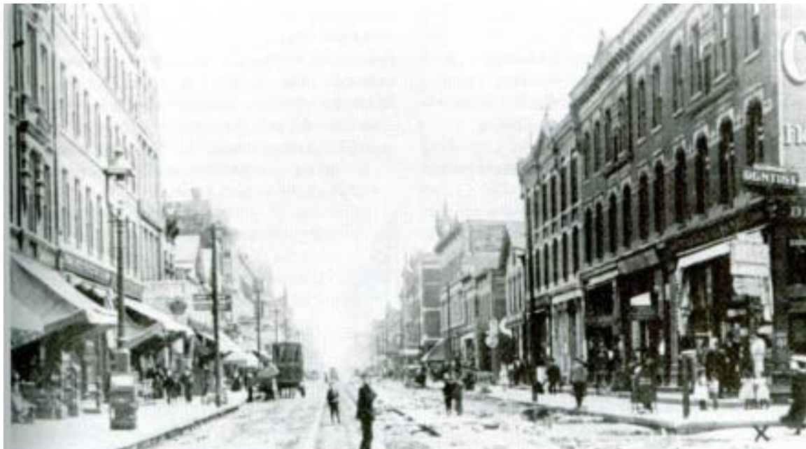
Commercial streetscapes and mixed-use buildings are a significant part of the history of Chicago neighborhoods. Two examples are Armitage and Milwaukee avenues. Top: Armitage Avenue looking east from Bissell in 1910 (from Chicago History Museum, reprinted in Terry Tatum, "Armitage-Halsted District."). Bottom: Milwaukee Avenue looking south from Evergreen in 1900 (from Elaine A. Coorens, Wicker Park from 1673 to 1979 , reprinted in Matt Crawford, "Milwaukee Avenue District.").
