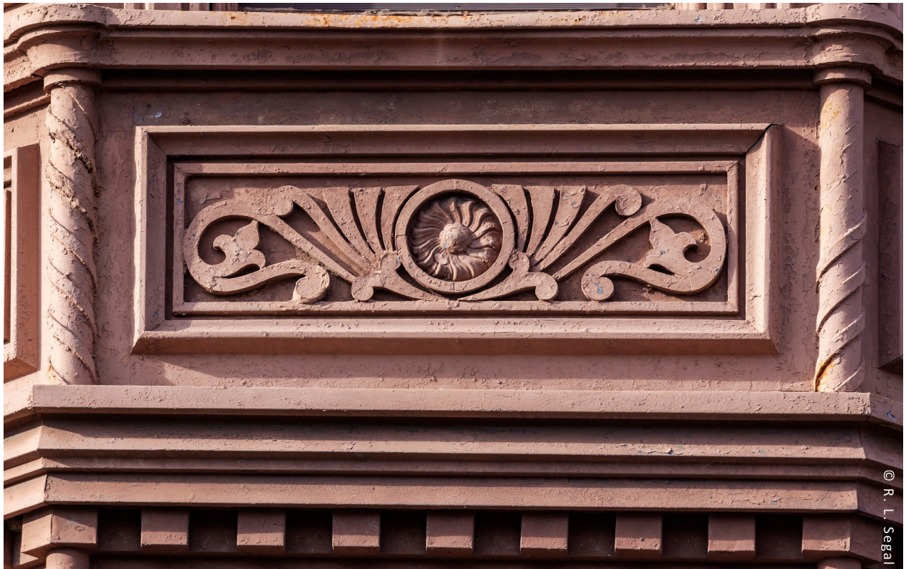
The building at 1730-1732 North Halsted Street is a fine example of the Queen Anne architectural style, with Romanesque Revival embellishments. Bottom: A detail of one of the building's pressed-metal oriel bays.
