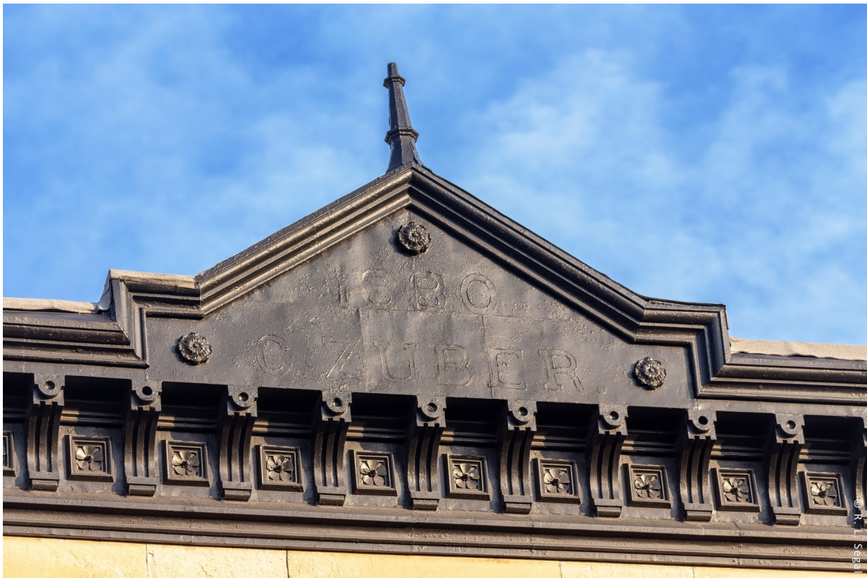
The buildings at 1727-1729 and 1733 North Halsted Street (as well as 1800 North Halsted) are handsome examples of the Italianate architectural style, ornamented with stone, decorative brick and pressed metal. Bottom: The cornice of 1733 North Halsted.
