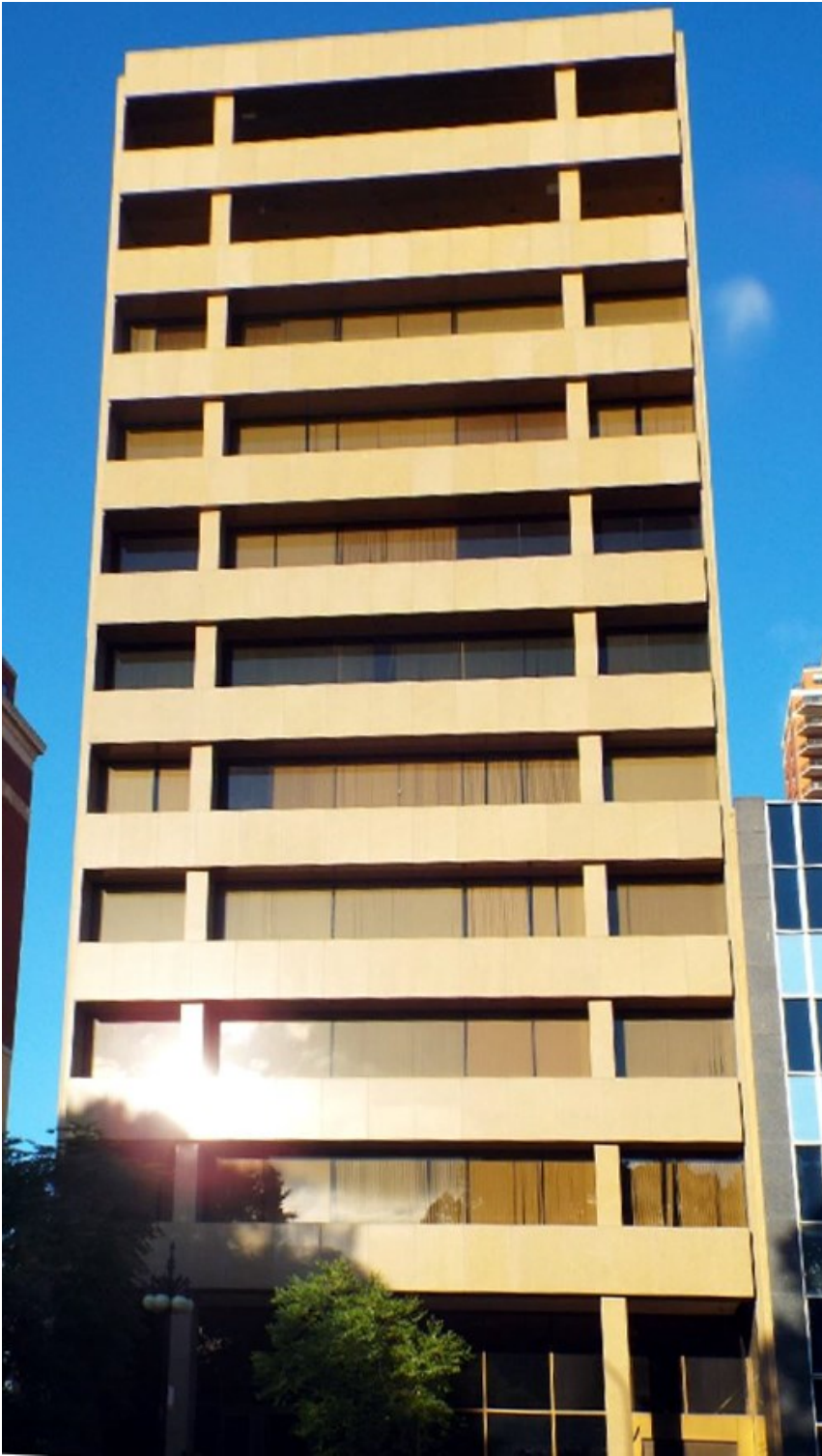
The Johnson Publishing Company Building's clearly expressed structure, rectilinear forms, open floor plans, and absence of ornament are hallmarks of the International Style. (EIDante C. Winston)
