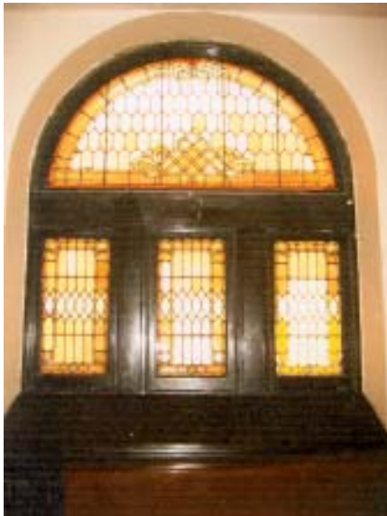
Interior details of the Metropolitan Apostolic Community Church Building. Clockwise from top left: View from the sanctuary's first floor looking south towards the church's semi-circular gallery; Gilt detail on the column capitals that support the upstairs gallery; Foliated gilt detailing on the massive concrete columns that support the roof; Coffered woodwork under the stairs leading to the gallery; Stained glass window detail on the first floor of the sanctuary.
