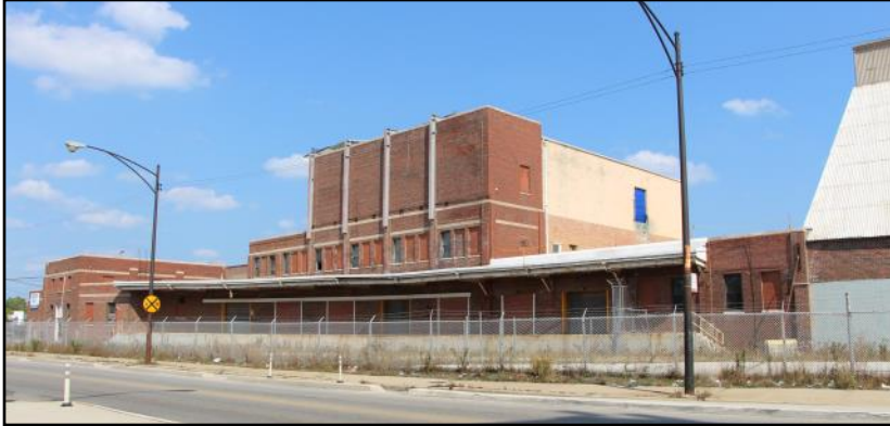
View of the west side of the Packaging Buildings along Elston Avenue. A covered curving dock accesses a railroad spur track.
