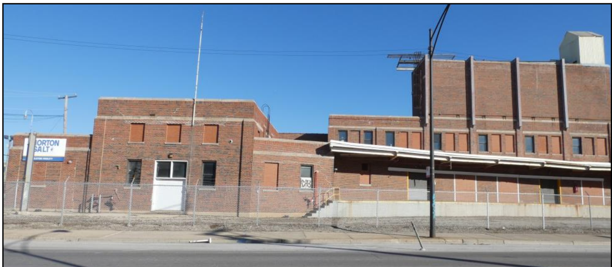
Along Elston Avenue, the Complex's Packaging Buildings are bordered by a rail spur track. At left is a boiler and power house, while the main packing and shipping section is to the right.
