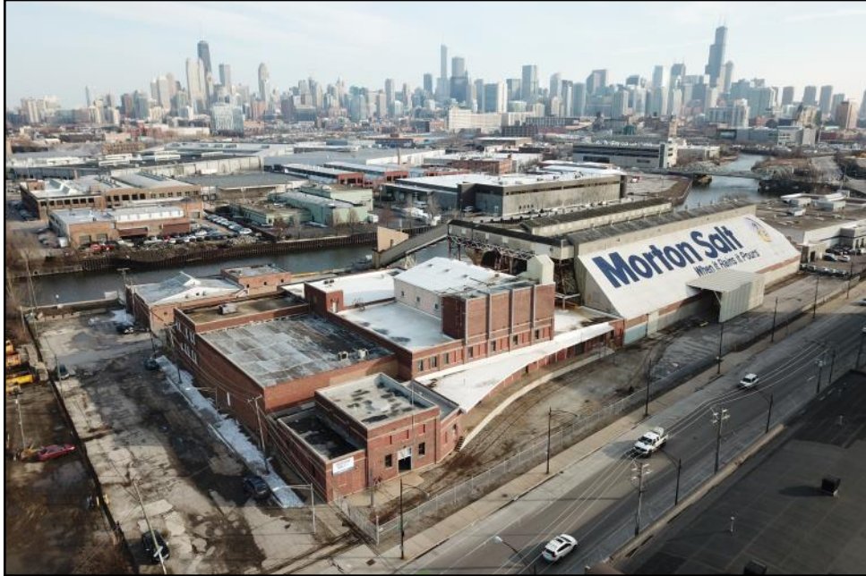
View of the Morton Salt Company Warehouse as it appeared in 2018 before the demolition of its original East Shed Building and enclosed conveyor system.
