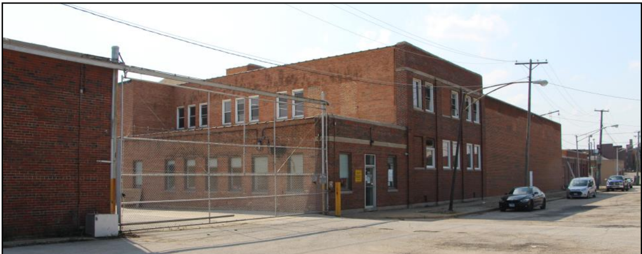
The main office, a two-story record storage block, and the 1968 (windowless) storage block of the Packaging Buildings face north onto Blackhawk Street. The Garage Building is at the far left.
