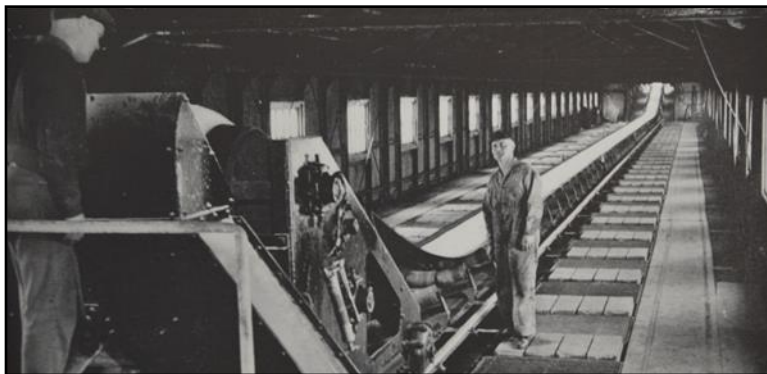
Above, salt was carried along internal conveyers in the roof of each shed. Workers could direct the salt into the shed at any point along the conveyer.
