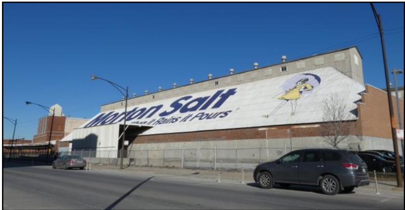
View of the west side of the West Shed Building with its distinctive painted roof that advertises the Morton Salt Company with its motto "When it Rains it Pours." The iconic umbrella-toting Morton Salt Girl is also shown.
