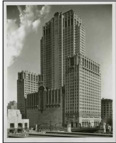
The Civic Opera Building (1927-1929, a designated Chicago Landmark). Midwest Manuscript Collection, Newberry Library.
