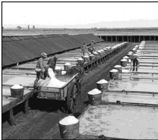
Above, workers collect salt in buckets from evaporating pans at a solar salt field near Syracuse, New York, circa 1900.
