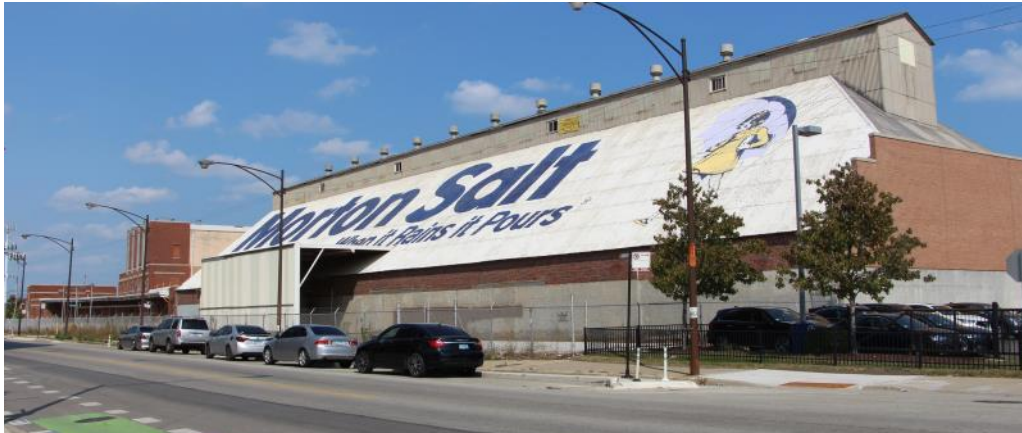
Left: The West Shed Building used for the storage of bulk salt. The view above, taken in 2020, shows the roof monitor where the internal conveyor was located.
