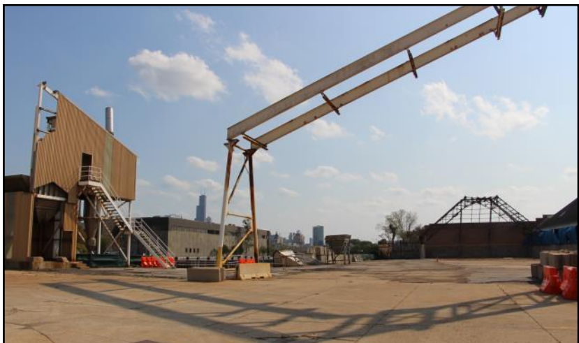
View looking south along the warehouse complex's Chicago River North Branch dock. At left is the former hoist, which pulled bulk salt from river barges. The metal frame that arches over the site once supported a covered conveyor belt that carried salt from the hoist to the East (demolished) and West Shed Buildings. The enclosed conveyor system and East Shed were demolished in 2020 due to structural damage.
