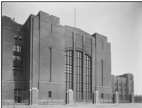
The firm also designed dozens of industrial buildings. Their designs typically embraced more utilitarian forms with simplified Prairie School-inspired details and forms. One example is the non-extant Crawford Avenue Generating Station built for the Commonwealth Edison Company in 1924. Chicago Photograph Collection, University of Illinois at Chicago.
