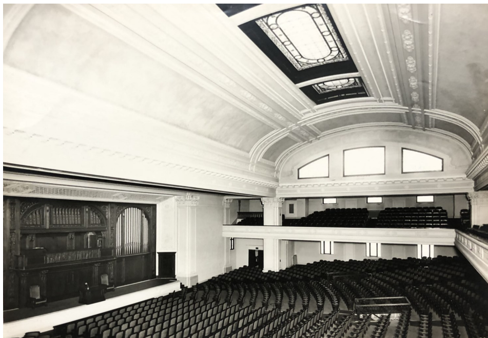
Designed for Chicago's Sinai congregation between 1909 and 1910 by prominent architect Alfred Samuel Alschuler, the Complex was dedicated in March of 1912. Upon completion, Alschuler had these photographs taken to document his work. The top photograph is looking southwest from the intersection of 46th Street and Grand Boulevard and shows the exterior of the synagogue and social settlement house, while the bottom photograph is of the sanctuary space (Chicago History Museum).
