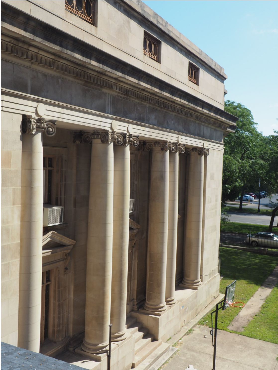
At the former Sinai Temple, Alschuler designed an impressively broad and imposing façade with a classical monumentality. Pictured here is the south façade of the synagogue which features the smooth limestone exterior, accentuated by a towering portico, pedimented fenestration openings, and dentil molding.
