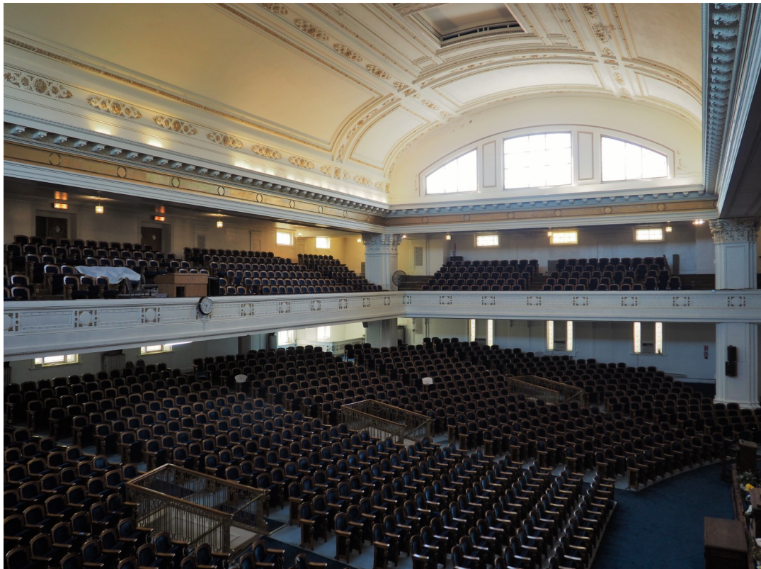
The former synagogue Complex was designed by the prominent and prolific Chicago architect Alfred Samuel Alschuler in 1909-1910 and completed in 1912. Pictured here is the exterior of the synagogue (top) and the interior sanctuary space (bottom).
