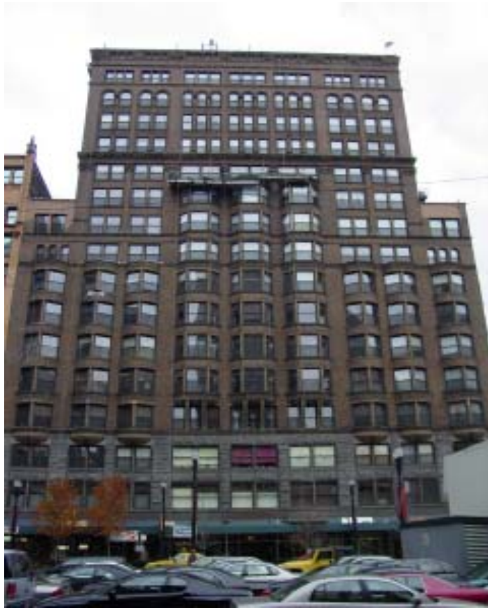
Jenney's earliest surviving skeleton-frame buildings are (below) the Second Leiter Building (built as a department store building and for years the Sears, Roebuck & Co. Department Store) at State St. and Congress Pkwy. and (right and above) the Manhattan loft manufacturing building at Dearborn St. and Congress Pkwy., both completed in 1891. Both are designated Chicago Landmarks.
