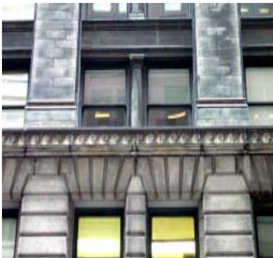
Right: The New York Life Building's upper floors clearly express the building's underlying steel frame through projecting piers and recessed spandrels. Above: The building's third floor is clad with rusticated granite. Attached columns ornament paired windows on upper floors. Top: The top floors are detailed with Classical-style moldings, pediments, and panels of foliate ornament.
