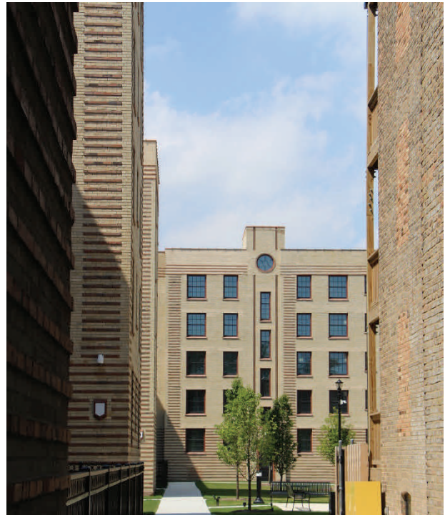
View from the street looking into the rehabilitated courtyard, 2017.
