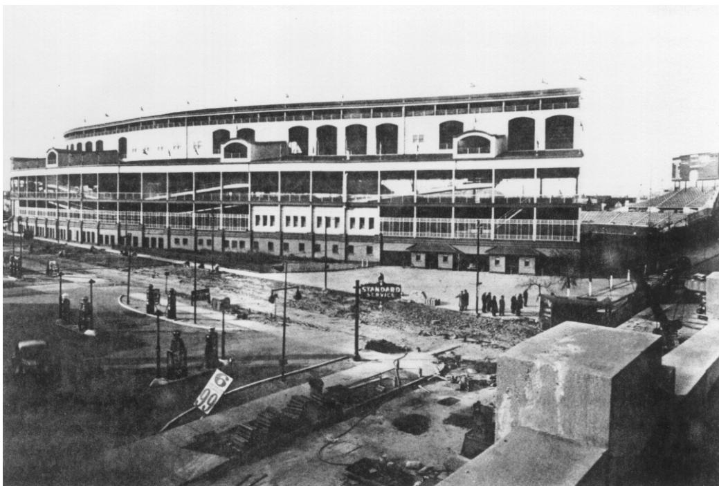
The ballpark's seating capacity at its opening in 1914 (top) was 14,000. After construction of the upper deck in 1927-28 and the outfield bleachers in 1937, capacity increased to more than 39,000. The above photo dates to the widening of Addison Street in 1939.
