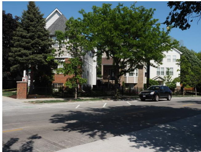
Development 'DP720 Zone B' North of Milwaukee
