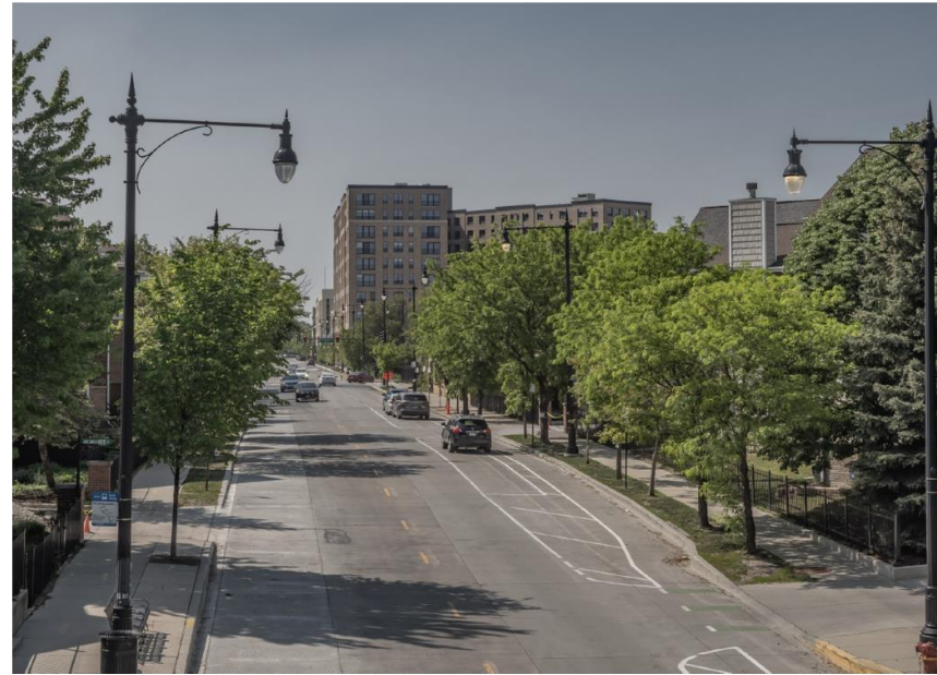
Milwaukee Ave - Looking NW
