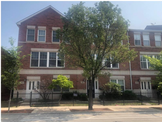
Development 'DP720 Zone B' North of Milwaukee
