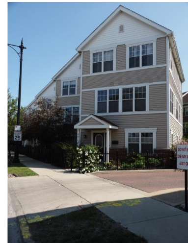
Development 'DP720 Zone A' South of Milwaukee
