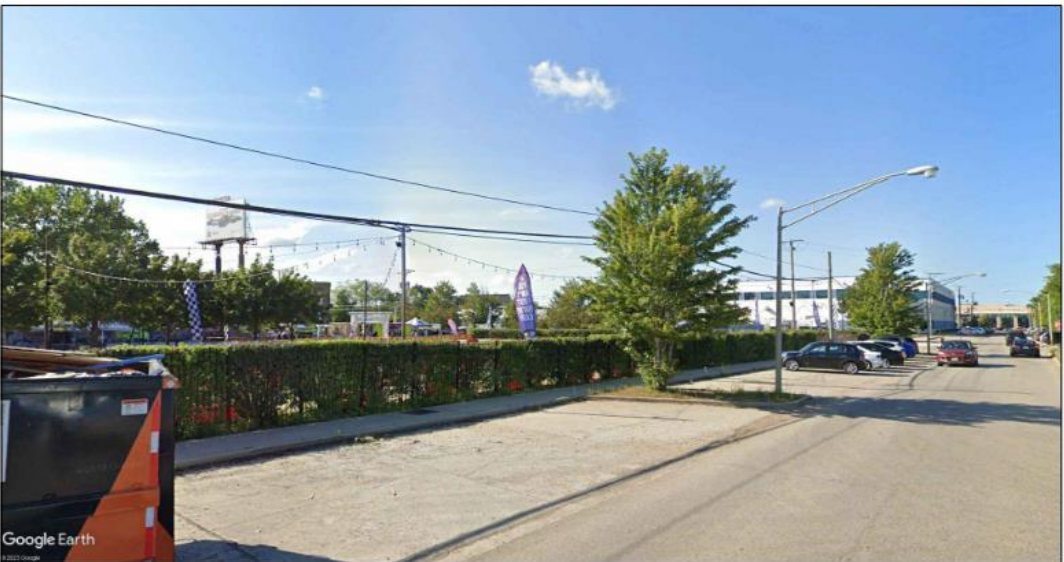
VIEW FROM SE CORNER ON MAGNOLIA AVE
