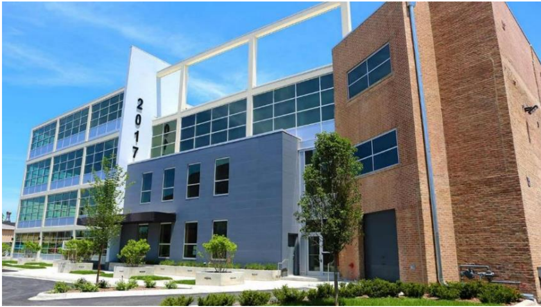
West Elevation Facing Mendell Street
