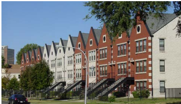
Three story townhomes line Bowen Avenue.
