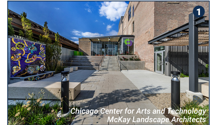
Enlarged entry plazas can be inviting both to building users and the broader public.
