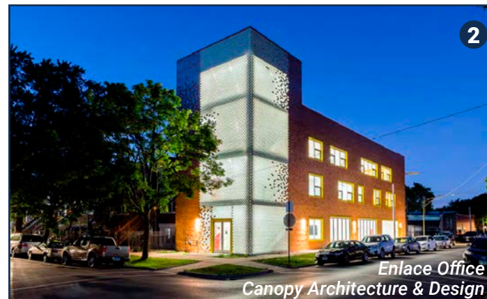
Enlace Office Canopy Architecture & Design Operable glass panels provide natural light and integrate with the brick to offer a defining feature at the corner.
