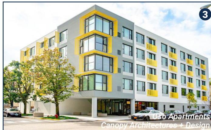
Setting back building entrances at corner sites address both the primary street and the side street.
