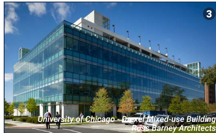
Wrapping structured parking with program (e.g. offices) shields unpleasant views and expands usable space.
