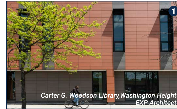
New terra cotta rainscreen curtain wall replaced a hazardous uninsulated brick façade.
