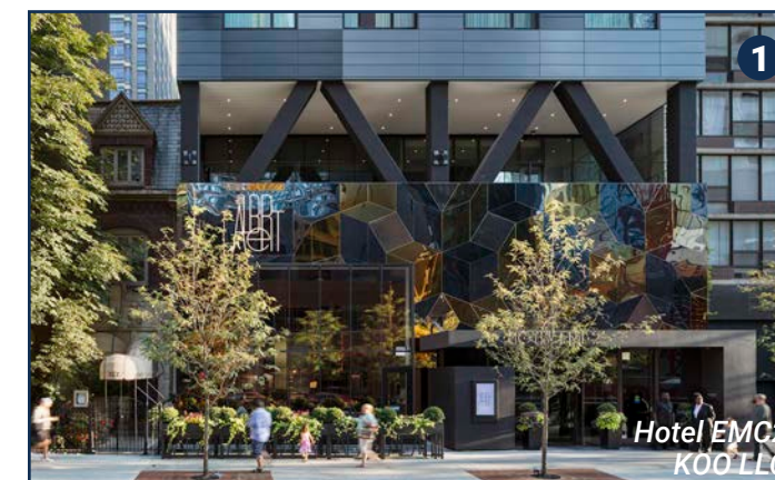
Stainless steel in three colors are used to create a colorful, sculptural, and inviting entrance.
