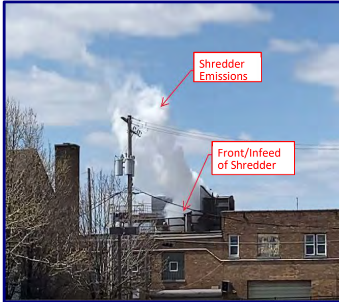
Figure 2 – Typical Uncontrolled Exhaust from Front/Infeed of the Hammermill Shredder at SIMS South Paulina
