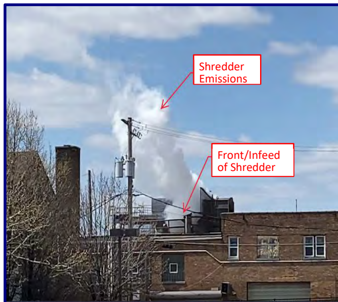
Figure 1 –Uncontrolled Exhausts from Shredder Raw Material Inlet SIMS South Paulina
