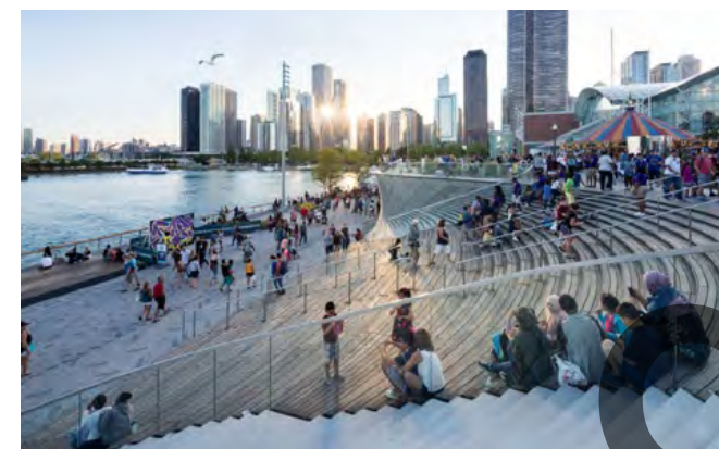
WAVE WALL AT NAVY PIER - CHICAGO, IL 2.0 ACRES WIDTH OF STEPS: 50-90 FT
