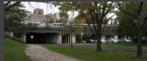
59 th /60 th Street Viaduct; 1893
