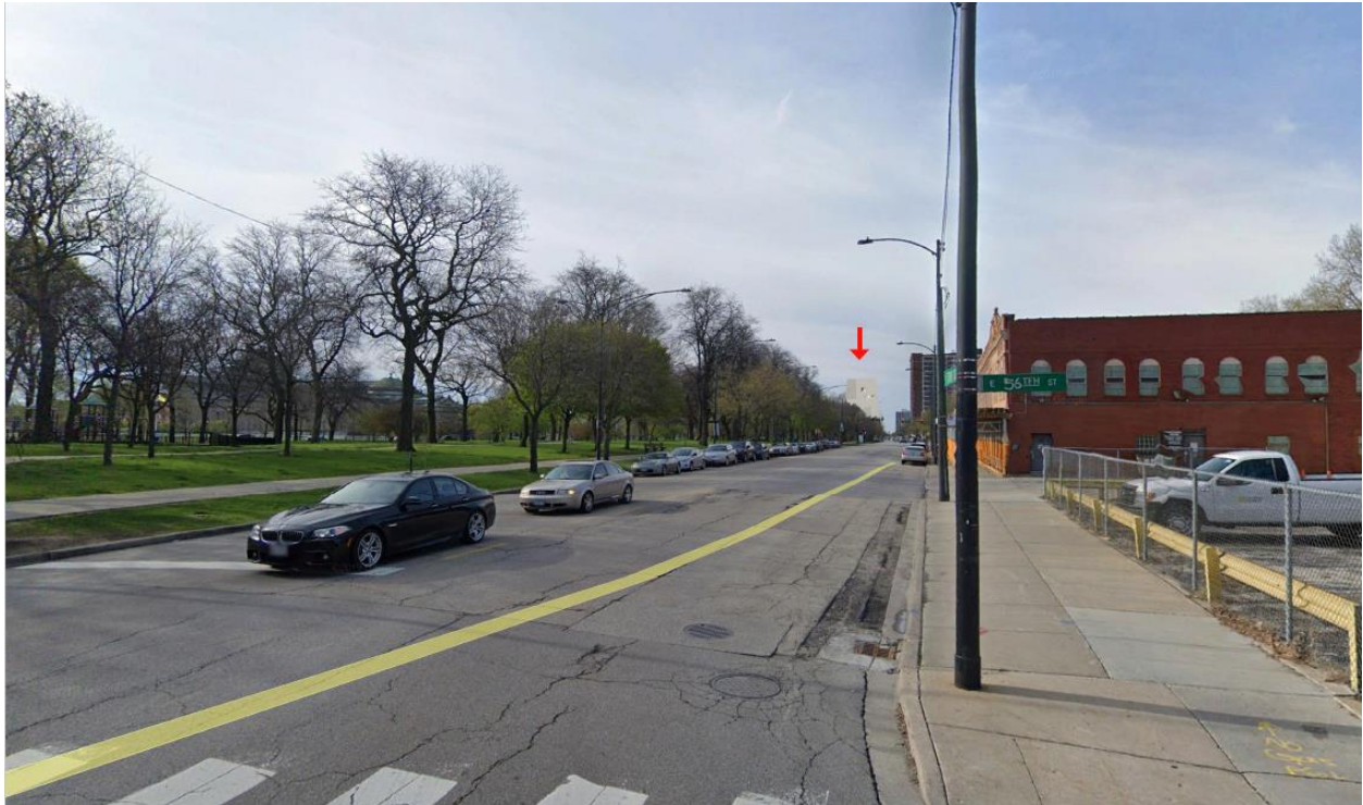
Photo 15: Streetview simulation from 56 th Street/Stony Island Avenue (Bret Harte Elementary School, Hyde Park East Historic District) southeast towards the OPC Museum building
