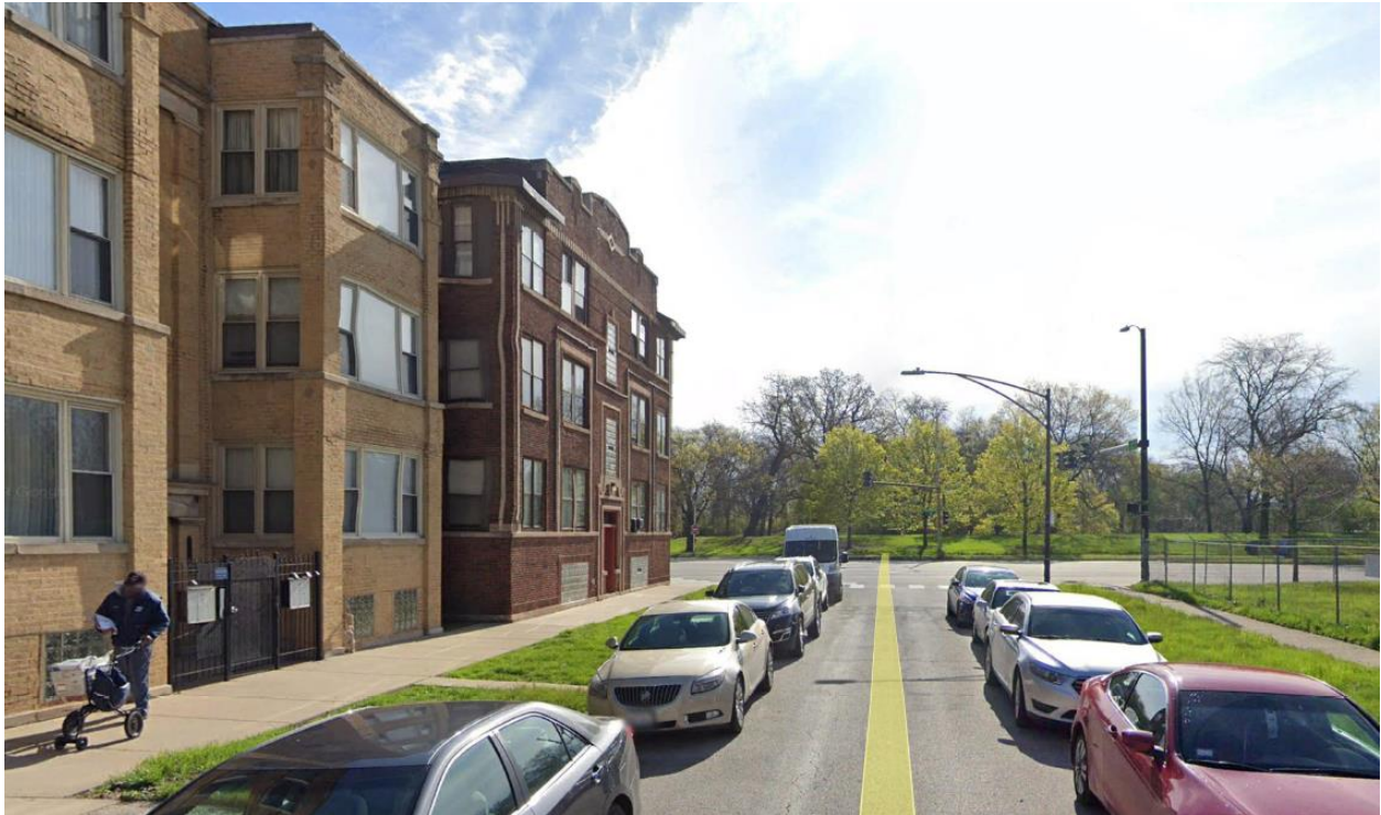
Photo 7: Streetview simulation from William Dexter Three-Flat northeast towards the OPC Museum building (Not Visible at street level)
