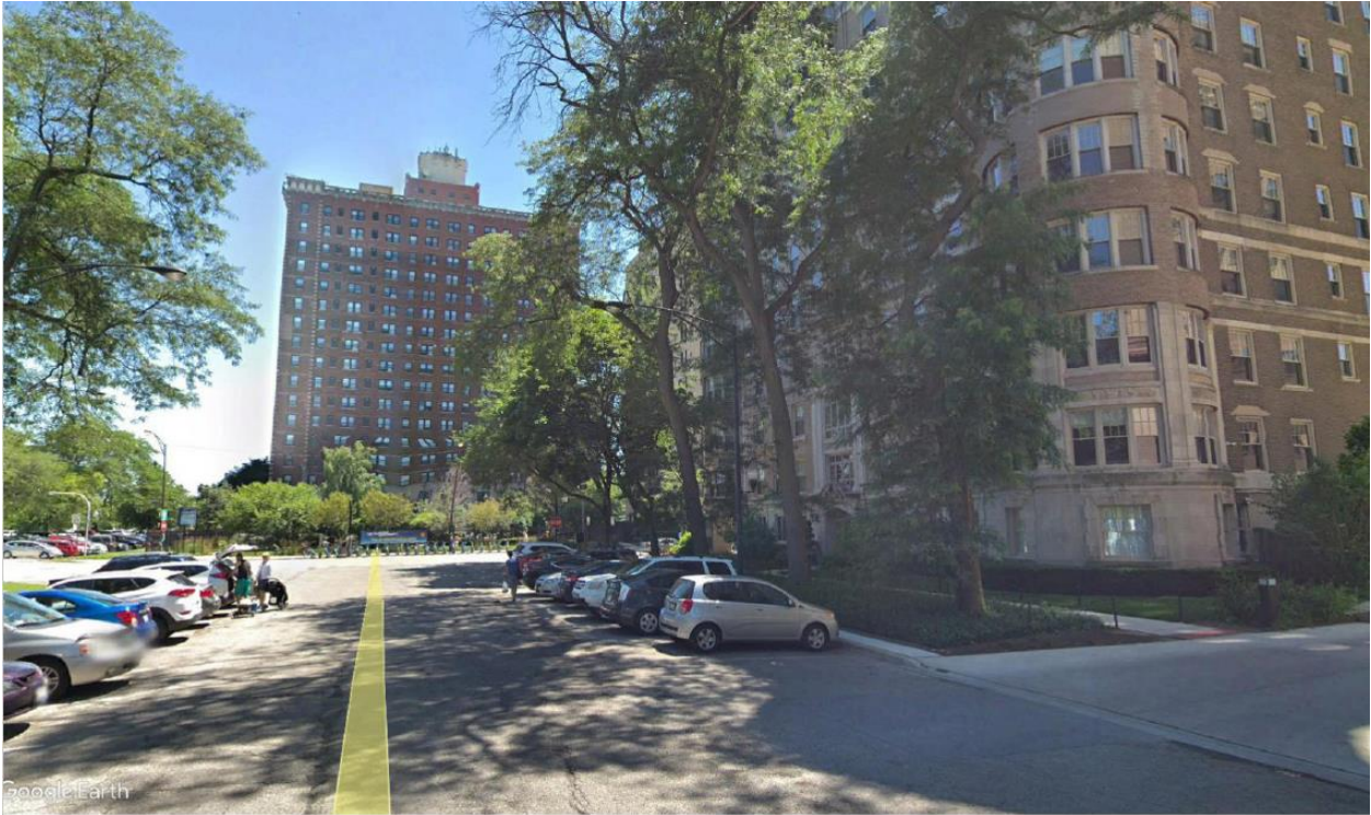
Photo 18: Streetview simulation from Jackson Shore Apartments, Shoreland Hotel (Hyde Park East Historic District) southwest towards the OPC Museum building (Not visible from street level)
