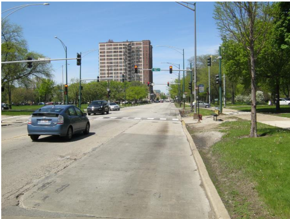
Photo 9: View from northbound Stony Island Avenue, south of 60 th Street, looking north
