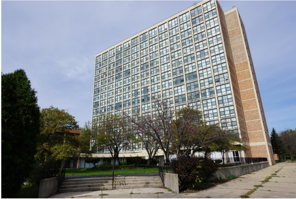
Photo 3: Jackson Park Terrace Housing Complex, 19-story Jackson Parkside Apartment high-rise, looking northwest from Harper Avenue toward south façade
