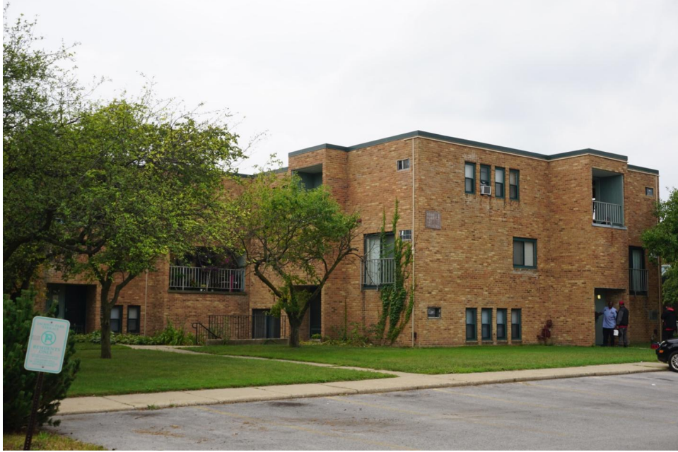
Photo 2: Jackson Park Terrace Housing Complex, three-story complex building, looking west from E. Public Way toward north façade
