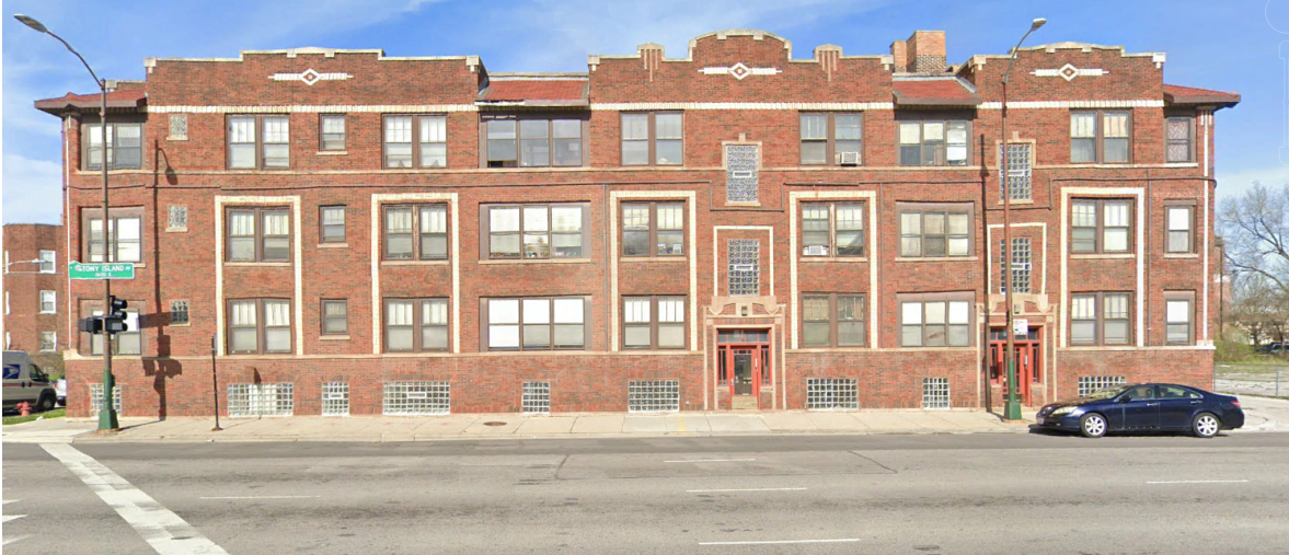
Apartment building at 6516-6520 S. Stony Island Avenue/1556-1558 E. 65th Place.
