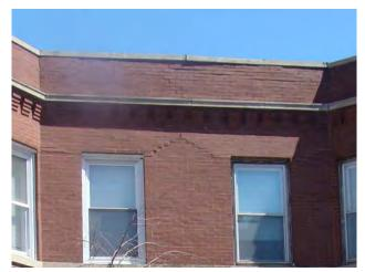
Step cracking in the brick on 5927/5929 Lafayette Avenue.
