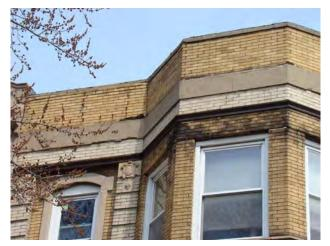
The concrete cornice is crumbling on 5841 Calumet Avenue.
