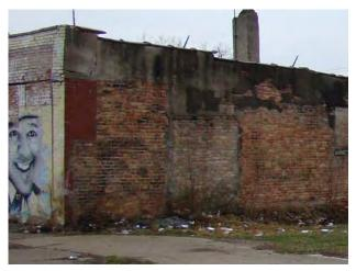
The rear wall of the previous commercial building is sagging and bricks have fallen out of the wall.
