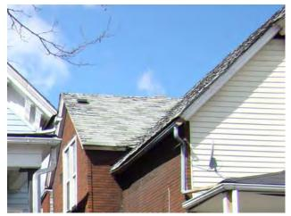
Deteriorated shingles on 5530 La Salle Street.
