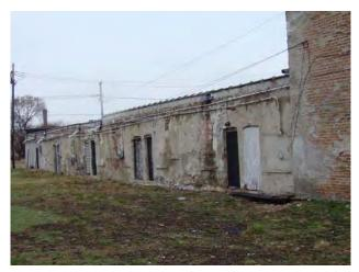
The rear brick wall of 221 East 58th Street is dilapidated.
