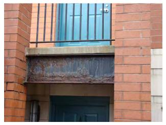
The steel beams used at this newer commercial development are rusted and deteriorated.
