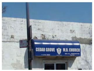
The church located at 5849 State Street has deteriorated bricks and mortar.
