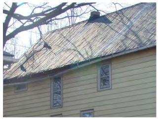
The gutter is falling off of 5957 La Salle. Note the roof is inadequately covered in roofing felt without the protection of shingles.
