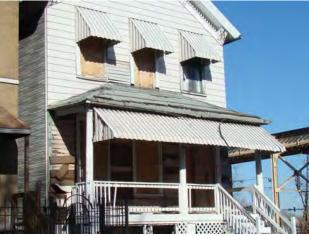
The porch roof on 5924 La Salle is deteriorated and the shingles have become dislodged.
