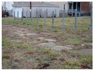
A sidewalk that has become overgrown and the concrete has crumbled.
