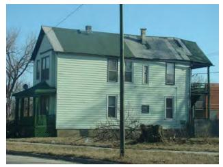
The roof on 5703 Lafayette Avenue is only covered in roofing felt. Note sagging rear porch roof.
