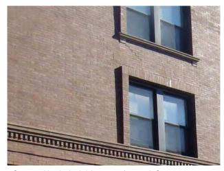
Step cracking in the bricks on 108/110 58th Street.
