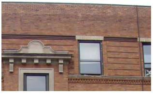
The parapet wall on 352 East 60th Street is in need of tuck-pointing.
