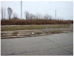
A deteriorated sidewalk along LaSalle Street.
