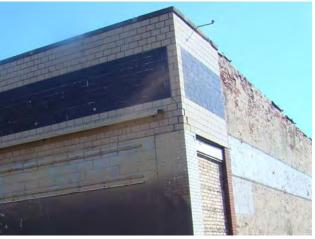
Step cracking and spalling in the brick walls of 5915 Michigan Avenue.
