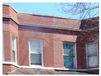
Step cracking in the brick of 5931/5933 Lafayette Avenue.
