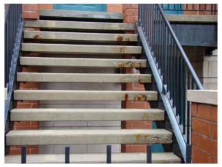
The concrete reinforcing inside of the steps is rusted due to moisture penetrating the concrete..
