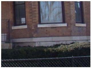
Step cracking in the bricks of 5551 La Salle Street.
