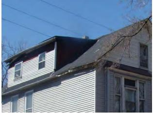
5924 Lafayette Avenue has dislodged siding, missing gutters sections and no shingles covering the roofing felt.
