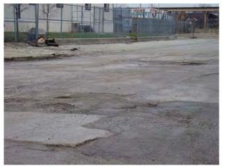
Deteriorated street paving located along 61st Street.
