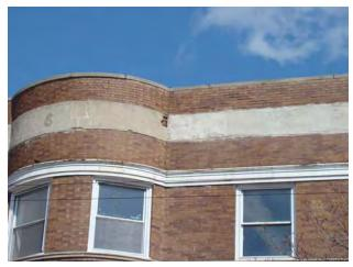
The bricks on 5632 Indiana Avenue are in need of tuckpointing. Note: concrete band is cracked and crumbling.
