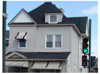
Roofing felt is being used to cover up a severely deteriorated roof on 5855 Indiana Avenue.
