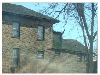
The roof is severely deteriorated and the gutter is falling off of 5821 Lafayette.
