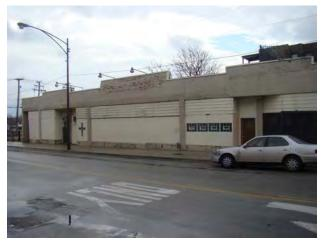
The parapet wall on 215 East 61st Street is leaning in and deteriorated.
