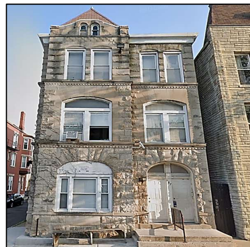
This 3-story walkup at 967 W. 19th St. is one of 15 affordable rental properties in the 15th, 22nd, 24th and 25th Wards that will be rehabbed by TRP.
